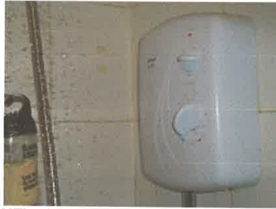
NEW SHOWER UNIT ABOVE BATH
