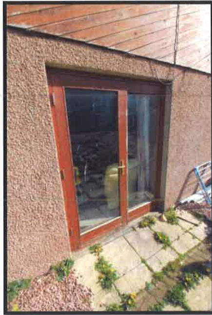
Figure 2 Lining Room French Doors - External.
