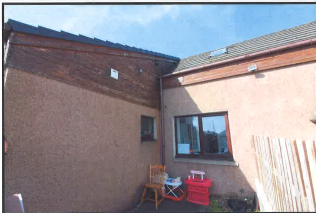
Figure 7- Main Bedroom and Kitchen windows, external.
