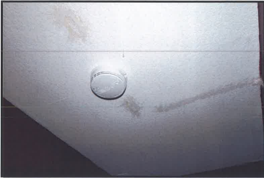
Figure 17 Inner Hall - Smoke alarm.
