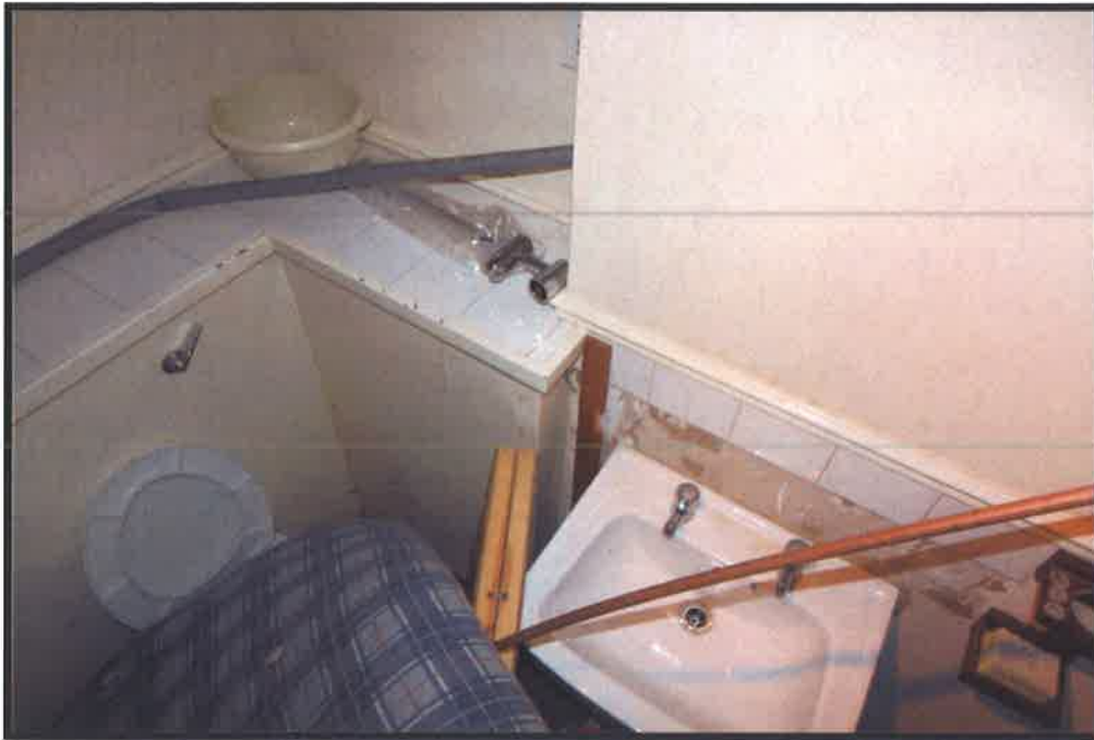
Figure 13 Main Shower Room - Overview of fittings.
