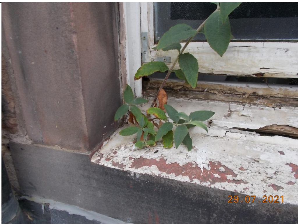
10. Detail of lower left section of Bathroom window from outside [Cill heavily decayed and vegetation established, lower sash patch repaired, cracked and missing pointing to joint between window and stonework]
