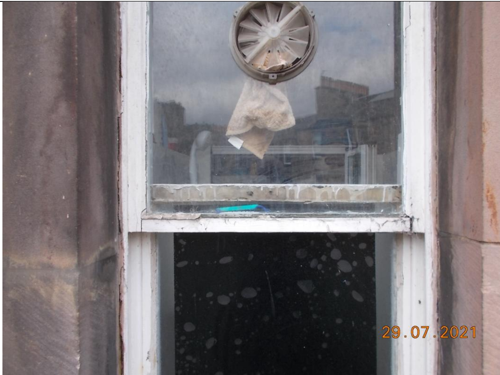
9. Detail of middle section of Bathroom window from outside [Missing and loose putty to upper glazing, open joints to lower part of upper sash, missing external cover to vent, cracked and missing pointing to joint between window and stonework]
