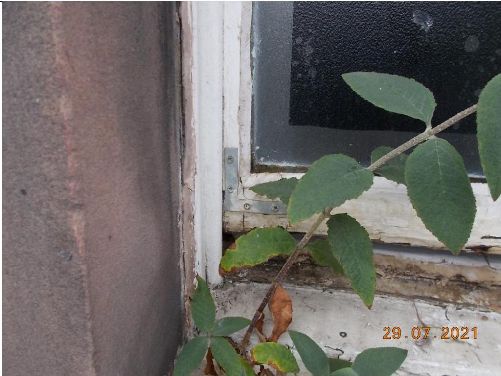
11. Detail of lower left section of Bathroom window from outside [Cill heavily decayed and vegetation established, lower sash patch repaired, cracked and missing pointing to joint between window and stonework]
