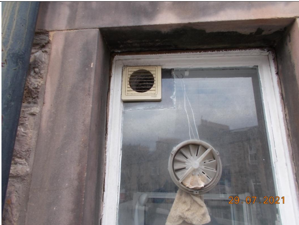
8. Detail of upper section of Bathroom window from outside [Missing external cover to vent, cracked and missing pointing to joint between window and stonework]
