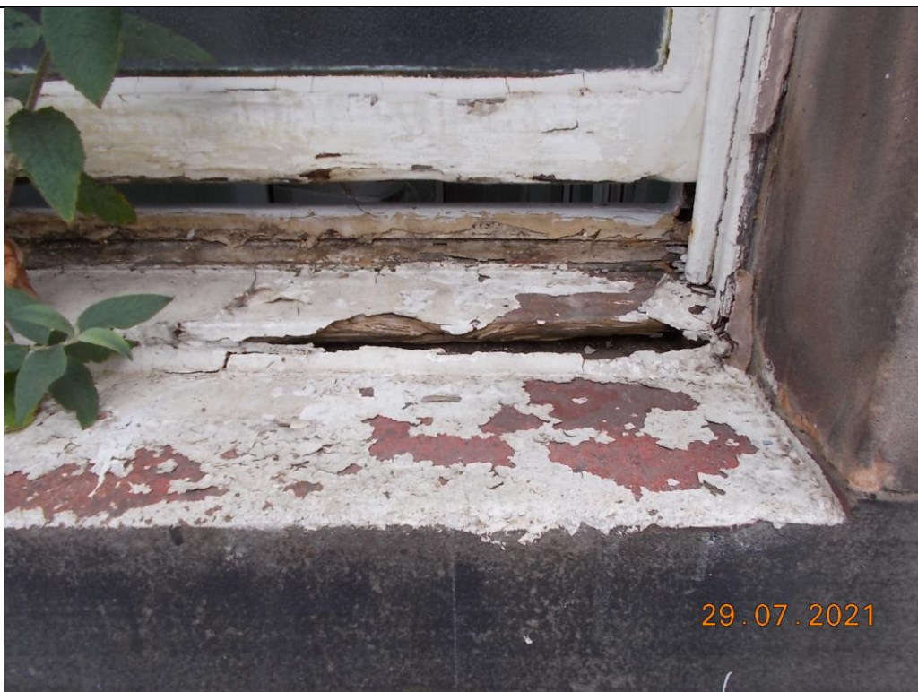
12. Detail of lower right section of Bathroom window from outside [Cill heavily decayed and vegetation established, cracked and missing pointing to joint between window and stonework]
