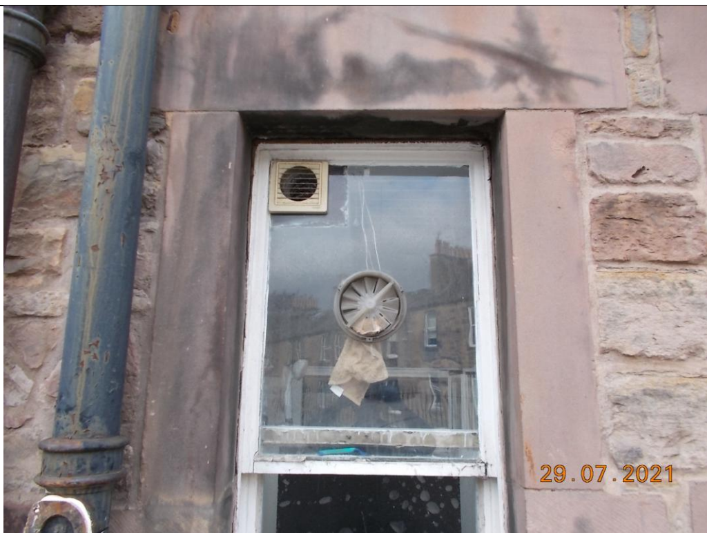
6. Upper section of Bathroom window from outside [Missing and loose putty to upper glazing, open joints to lower part of upper sash, missing external cover to vent, cracked and missing pointing to joint between window and stonework]
