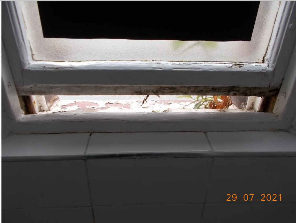
5. Detail of window cill and lower sash of Bathroom window from inside
