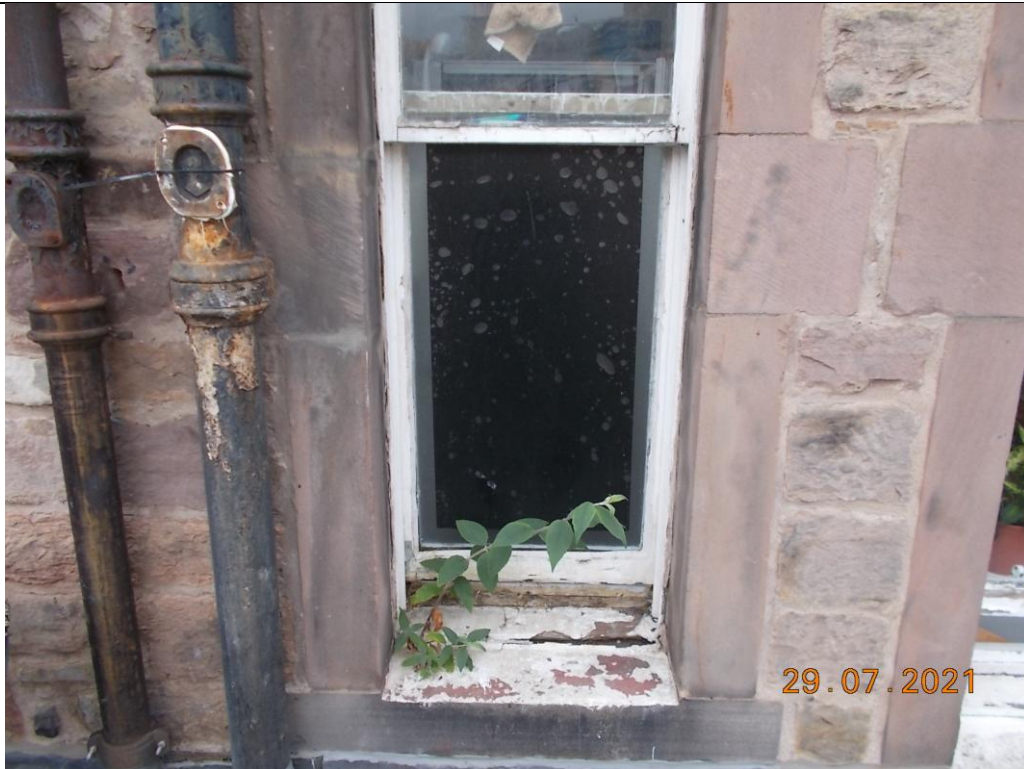
7. Lower section of Bathroom window from outside [Cill heavily decayed and vegetation established]
