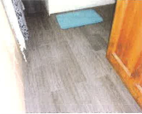
BATHROOM FLOOR COVERING
