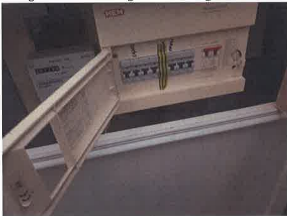
26 Consumer unit – cracked/damaged.
