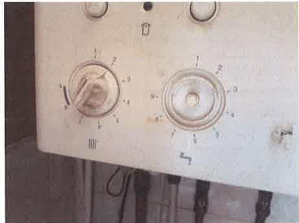
31 Damaged knob control.
