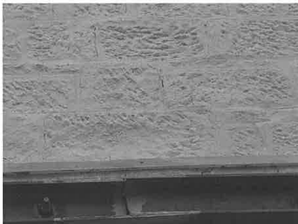
2 Cracking emanating above joint of steelwork restraint
