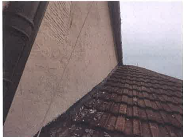
13 Poor render to rear elevation above roof (boss under tap test).
