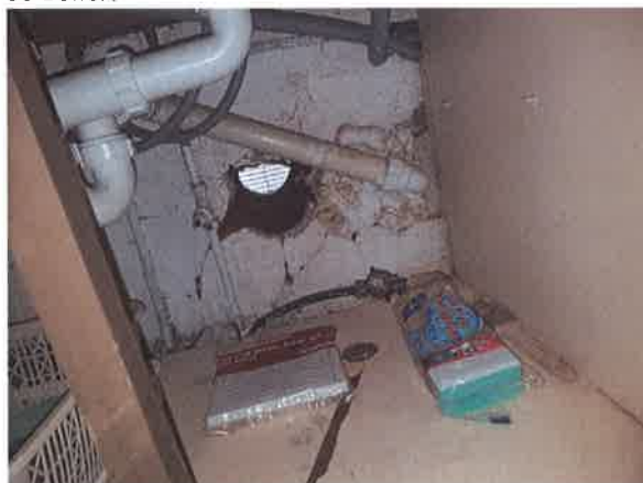
32 Vent and expanding foam below sink unit.
