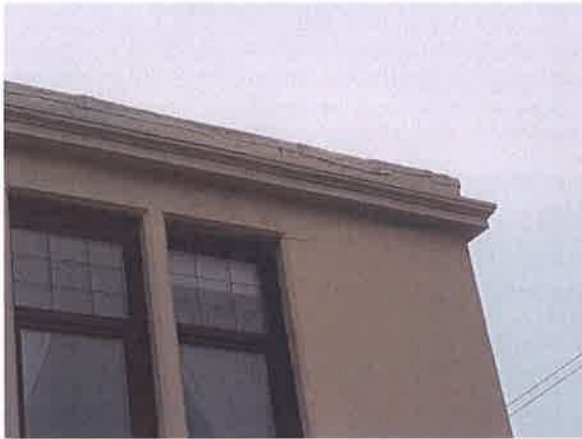
6 Uneven and poorly detailed lead to wallhead parapet.
