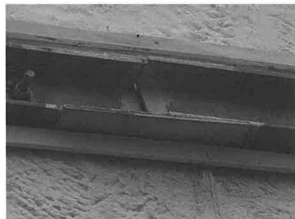
5 Joint of steel restraint.
