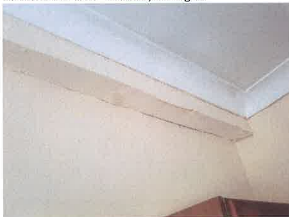
28 Water staining within Kitchen to boxing.
