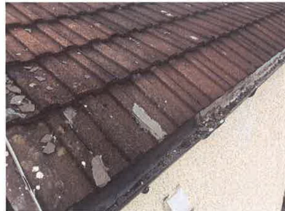
11 Interlocking tiles (patch repaired) to rear outshot.
