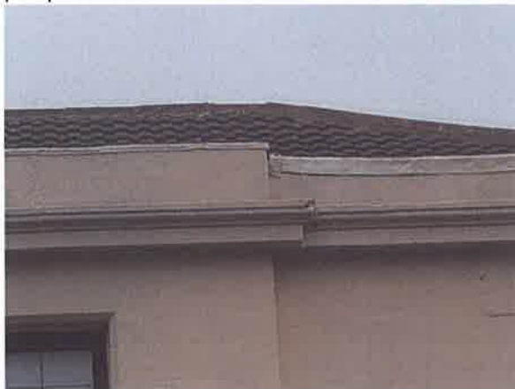
8 View of leadwork to wallhead and front roof pitch.
