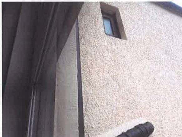
20 Cracking to render of Bathroom external wall.
