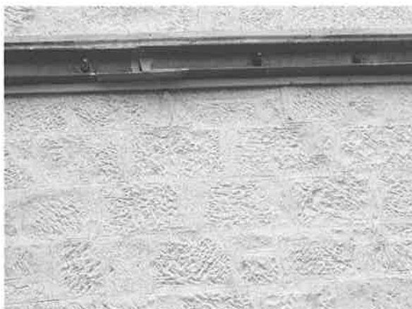
4 Further view of Gable restraint steel
