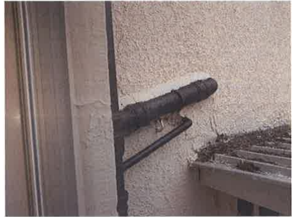
19 Cracking to render of Bathroom external wall.
