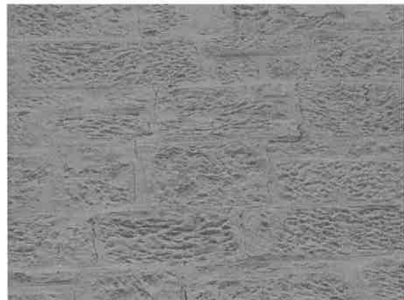
3 Stepped cracking to Gable Elevation.
