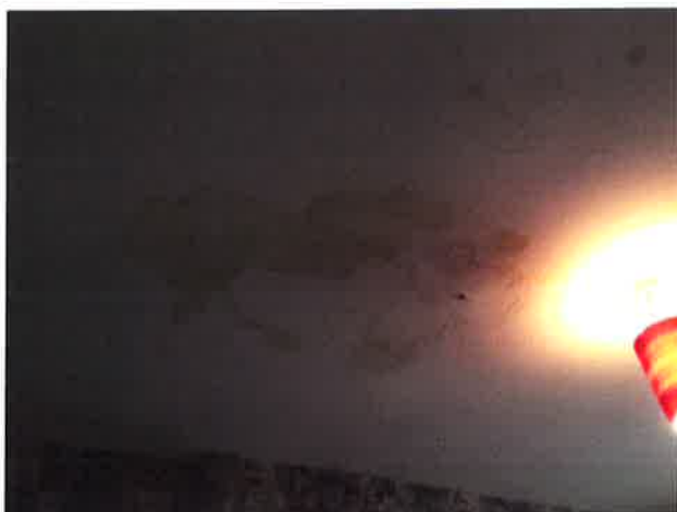
Bedroom 2 – south west – damp staining on ceiling above window
