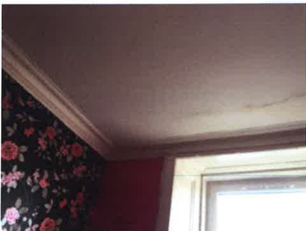
Bedroom 3 – north east – damp staining on ceiling in corner
