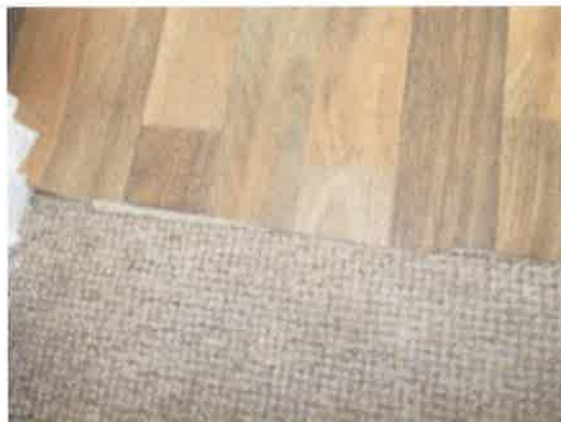
Bathroom Floor - loose fitting vinyl/no threshold bar.
