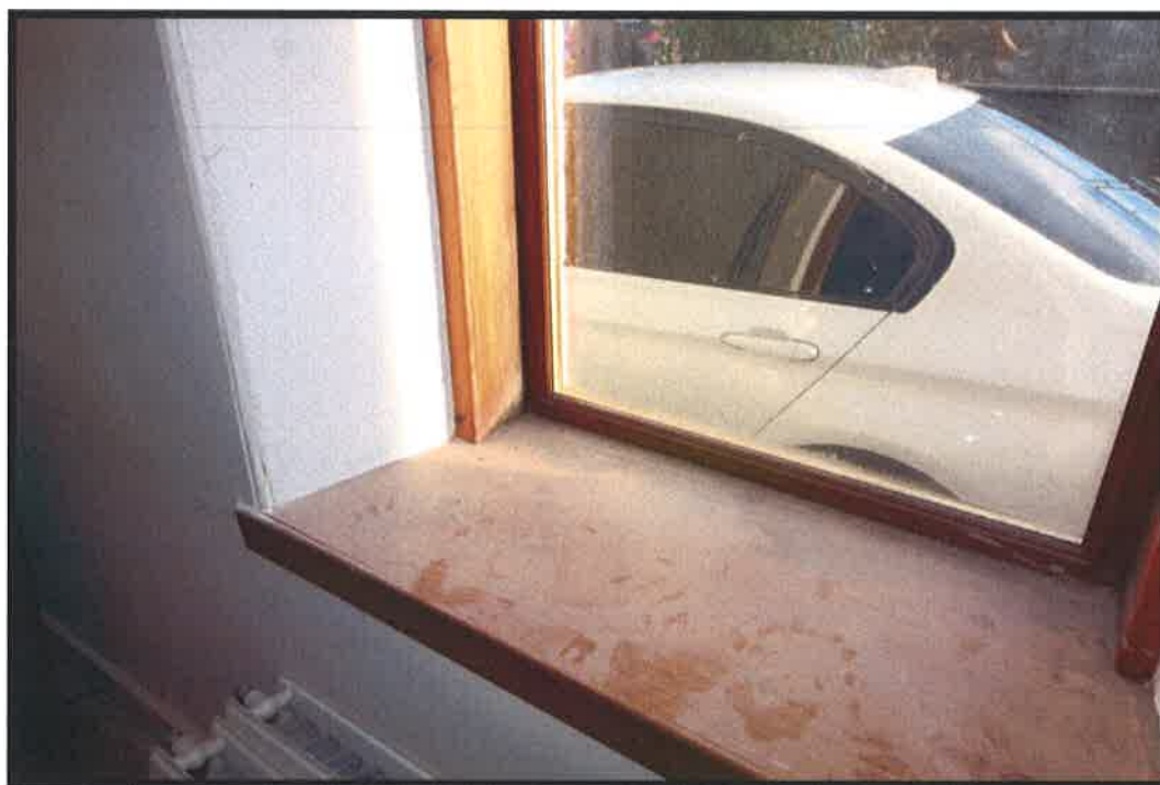
Figure 7- Middle bedroom - water marks to timber window sill.
