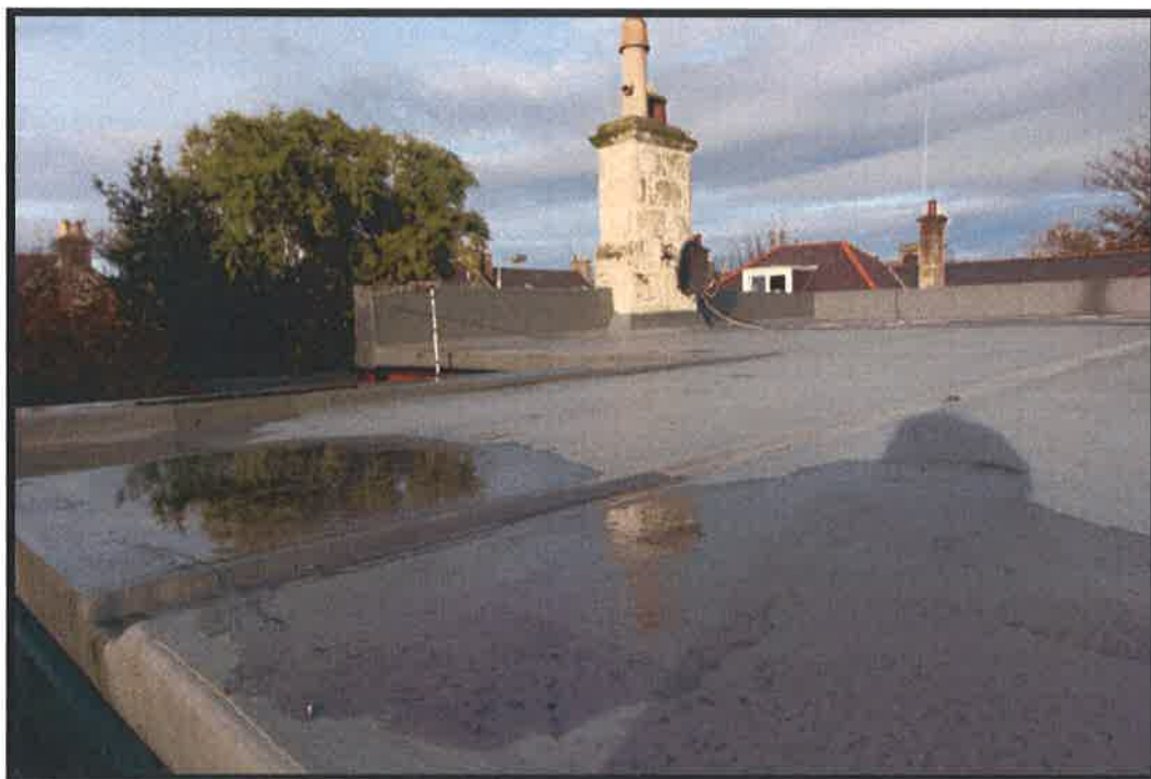
Figure 18 Rear section of flat roof with ponding over bathroom, as before.
