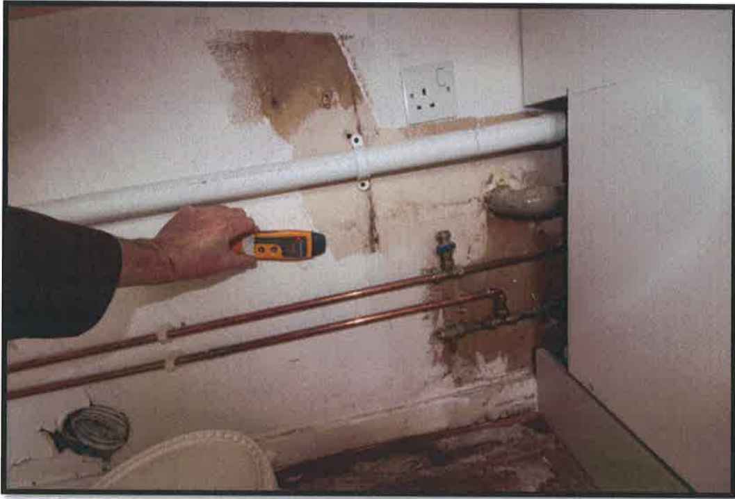
Figure 14 Former utility room/new kitchen - moisture meter reading (100%), as before.
