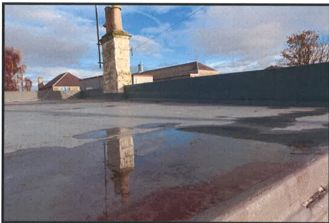
Figure 20 Rear section of flat roof at kitchen/utility room junction with ponding over former kitchen - as before.
