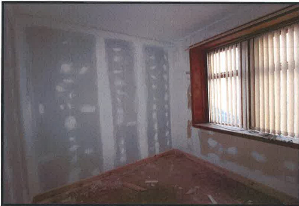
Figure 3 Front Bedroom -new plasterboard
