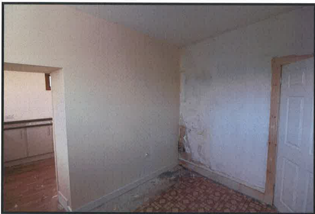
Figure 10 Former kitchen overview. Cabinets removed, linings part renewed.
