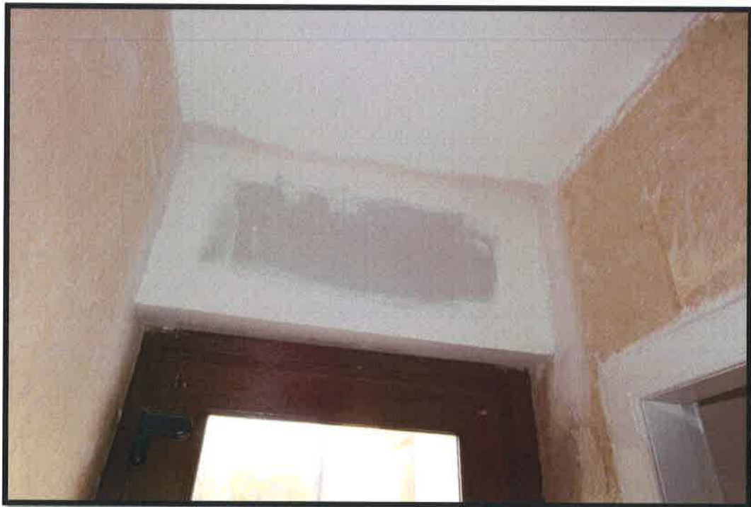
Figure 15 Rear hall - new plasterboard above rear entrance door.
