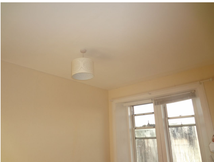
2. Bedroom walls and ceiling
