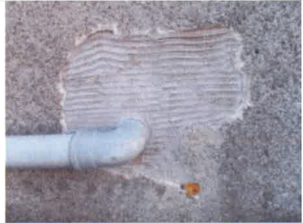
Front elevation - closer view of roughcast partial repair
