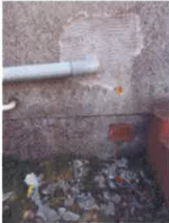
Front elevation - roughcast partial repair
