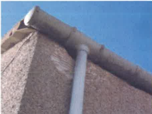
Front elevation - roughcast partial repair
