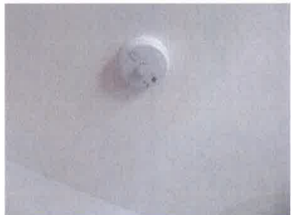
New ceiling mounted heat alarm in Kitchen
