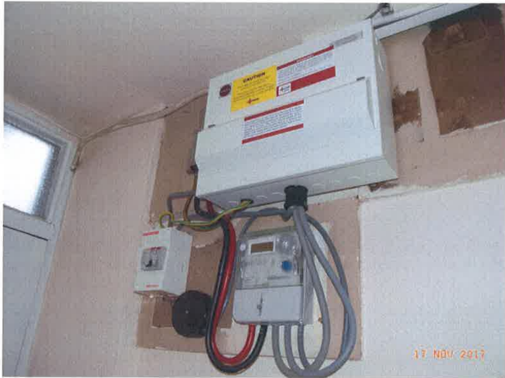
Electric meter and fuse box
