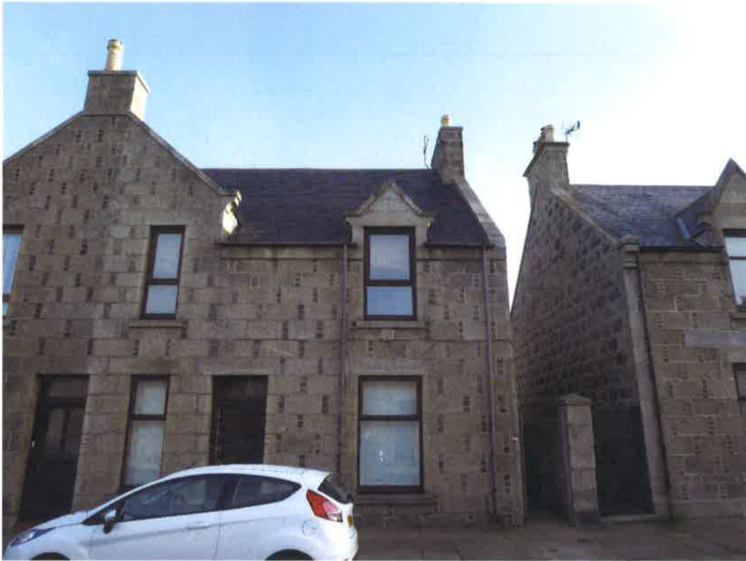
Front (Street) view – 1 st floor flat
