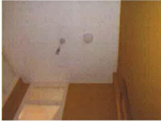
14. SMOKE DETECTOR IN UPPER LANDING
