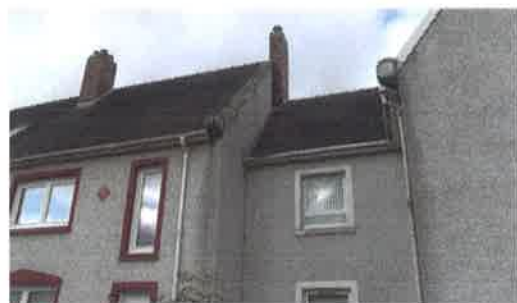
Photo 11 – Choked guttering
