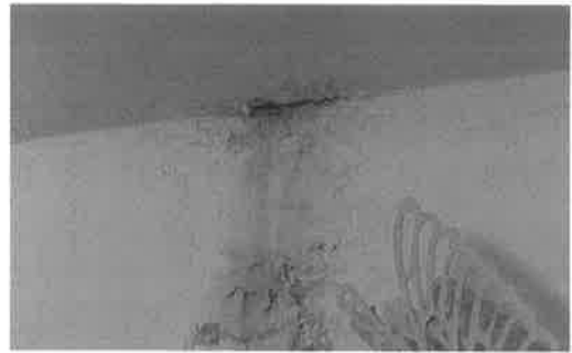
Photo 3 – Water damaged wall
