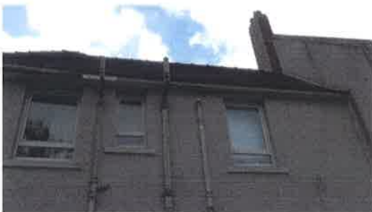
Photo 10 – Missing gutter/soffit
