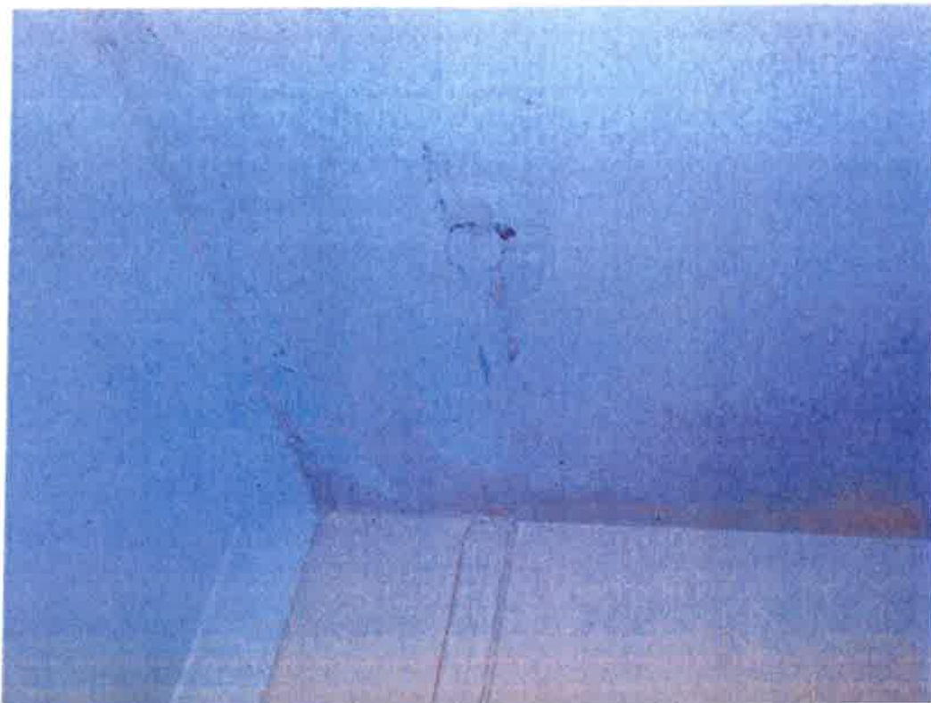
Flaking and peeling plaster and paint – high level sitting room
