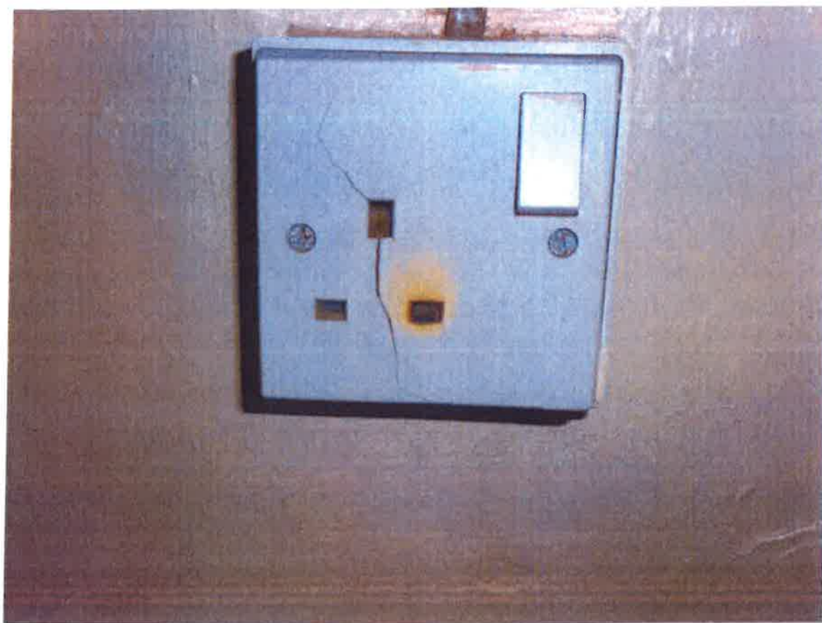
Defective broken socket in kitchen – signs of scorching
