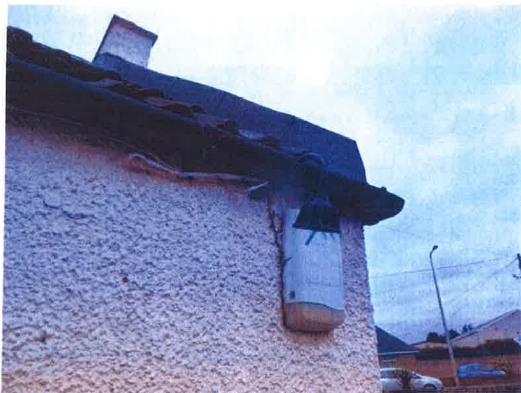
Defective light fitting at rear
