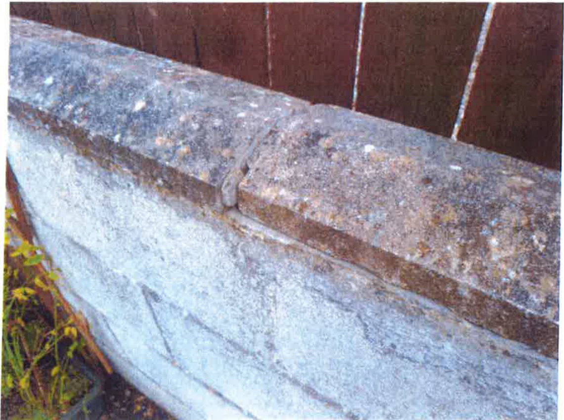
Loose coping stones to wall at rear
