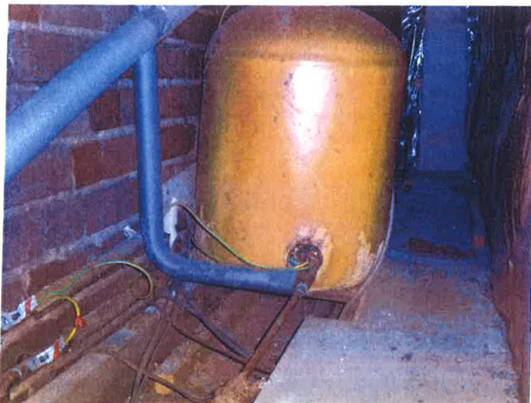
600mm x 450mm hot water cylinder to loft area
