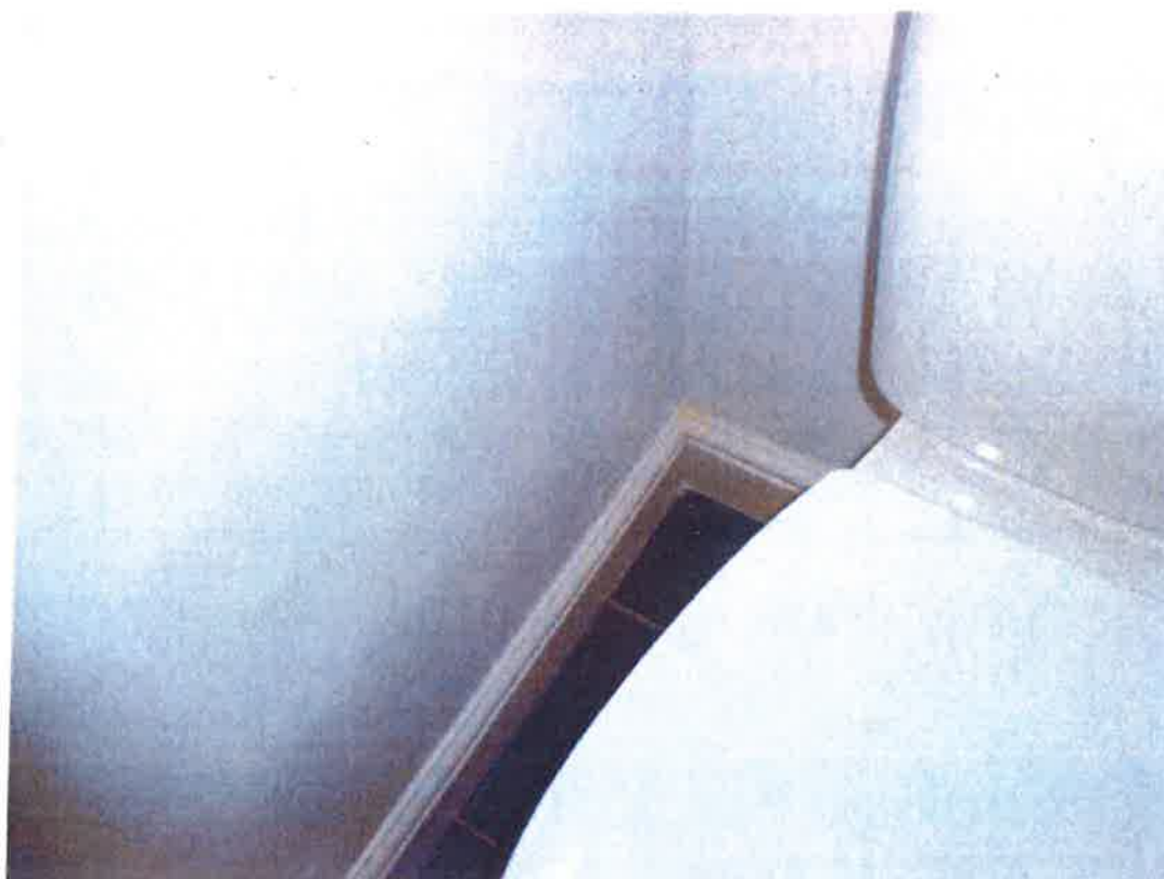
Wet area inside bathroom at low level – only around WC bowl
