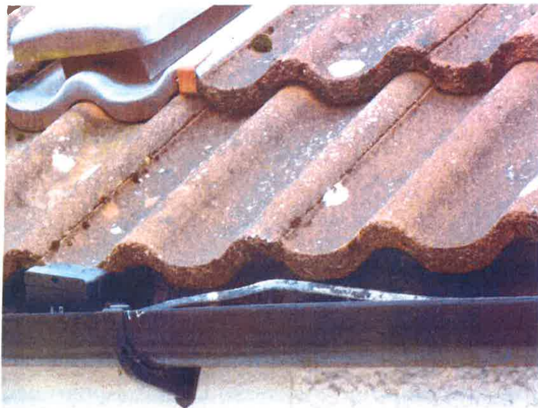
Cable in gutter at rear
