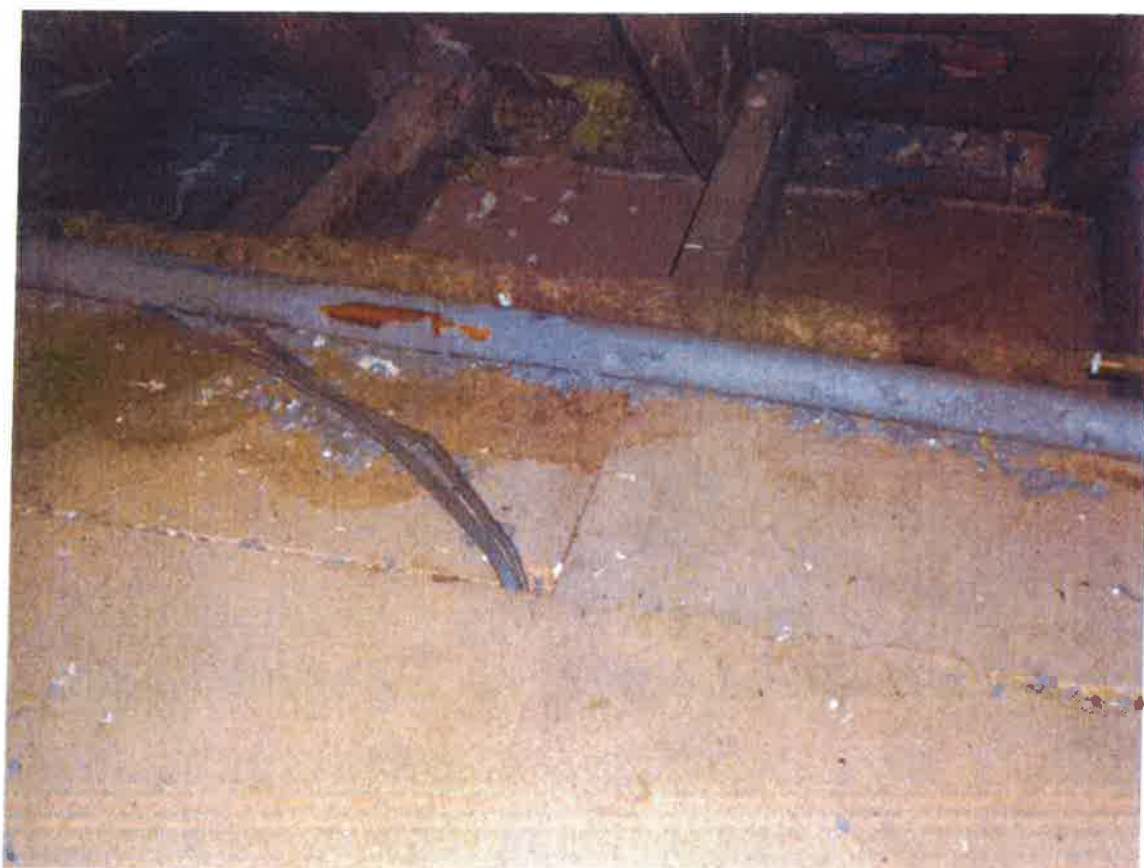
Rodent and vermin damage to loft space
