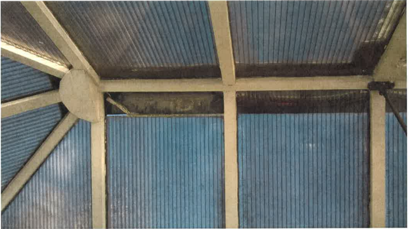
3d) Left slipped glazing panels exposing the flashing with gap to open air
