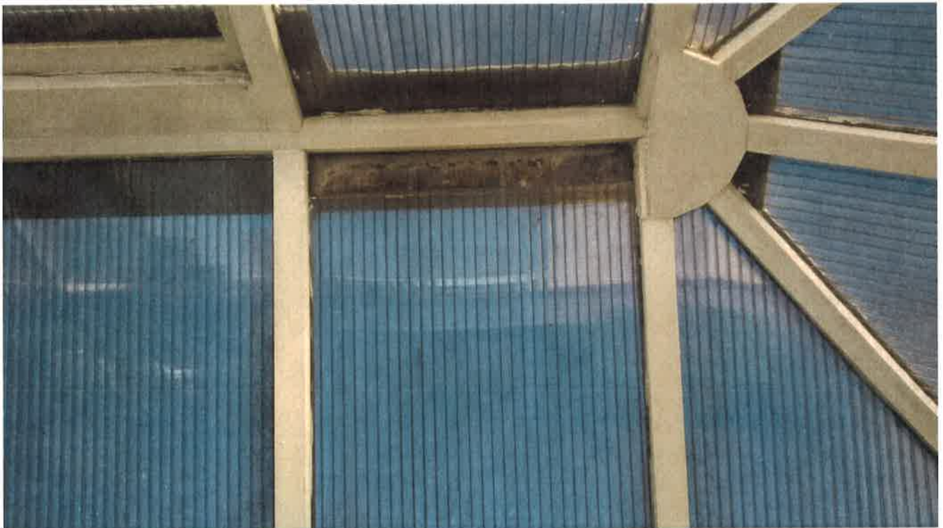
3e) Right slipped glazing panel exposing the flashing
