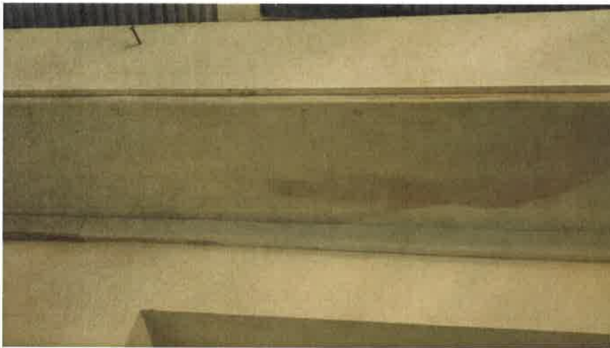
3b) Internal evidence of water penetration beneath valley gutter
