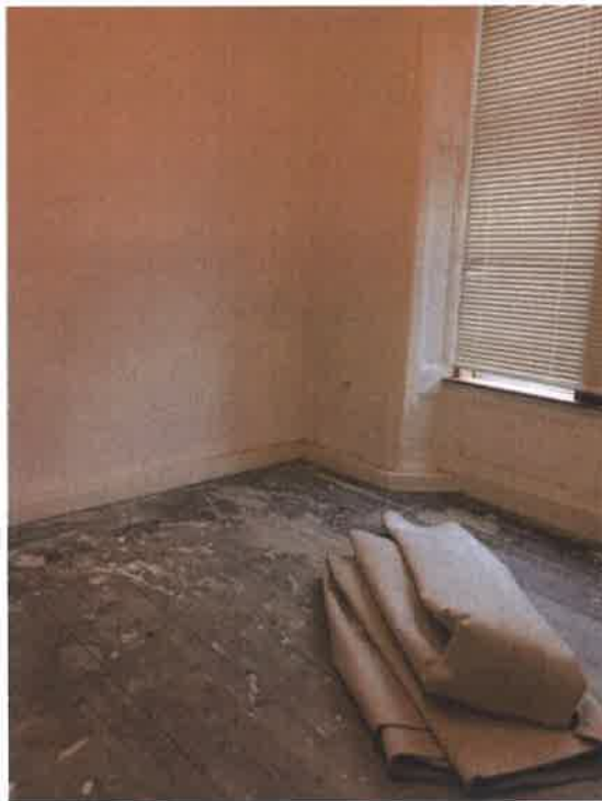
Photograph 10: Bedroom: general view
