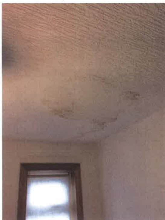
Photograph 3: Kitchen: ceiling - staining
