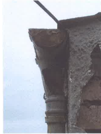
8 & 9 illustrate broken and defective joint at boiler-house door
