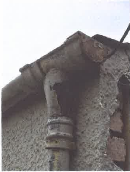
8 & 9 illustrate broken and defective joint at boiler-house door
