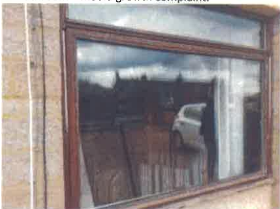
17 External view of Living Room window.
