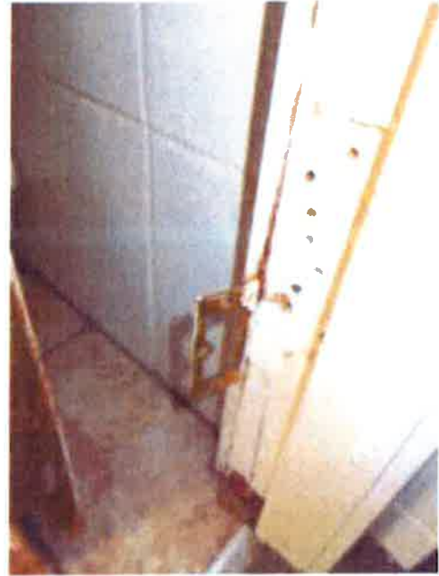
Bathroom door - damaged lower hinge
