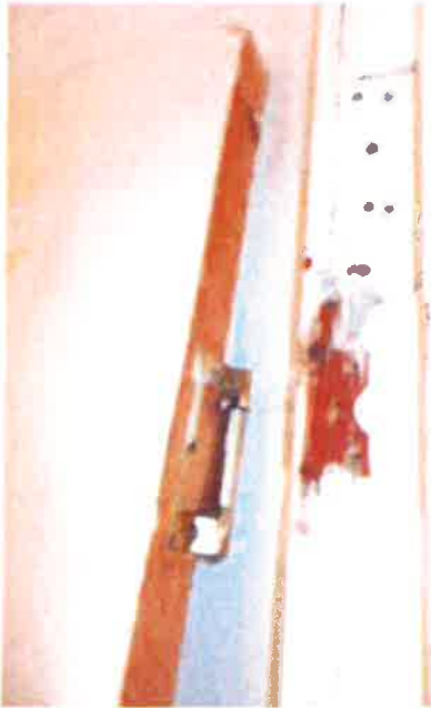
Bathroom door - damaged upper hinge
