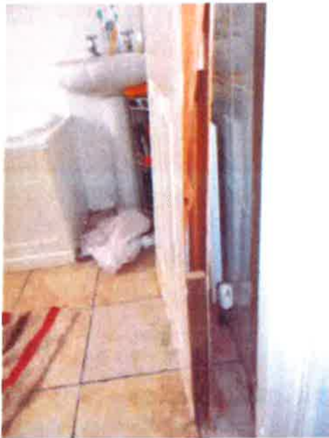
Bathroom door - damaged/exposed core and detached from hinges
