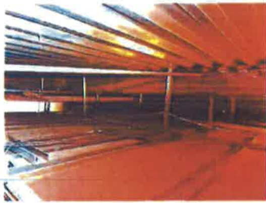
6, 7 & 8:- Void above ceiling immediately below profile steel roof decking
