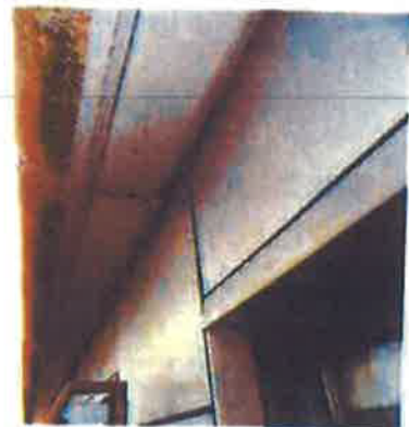
3. Defective "soffit" joint (eaves)
