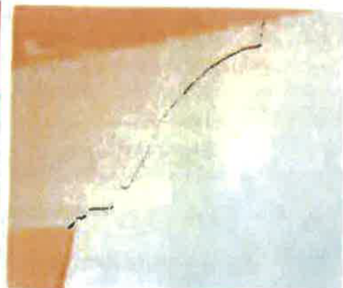
4 & 5. Cracking above right hand corner of front facing window
