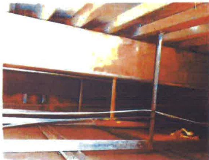
9. Insulation at external wall in void over ceiling
