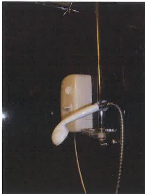
10. Bathroom shower showing loose bracket on riser
