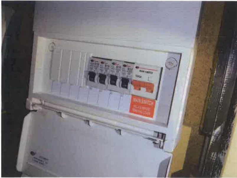
17. Distribution board – main switch
