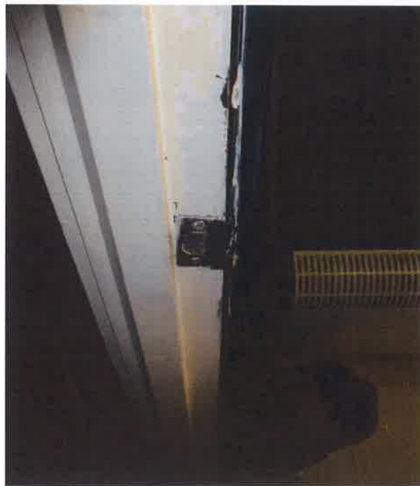
14. Bathroom showing panel heater and trim at wall boarding interfering with door catch
