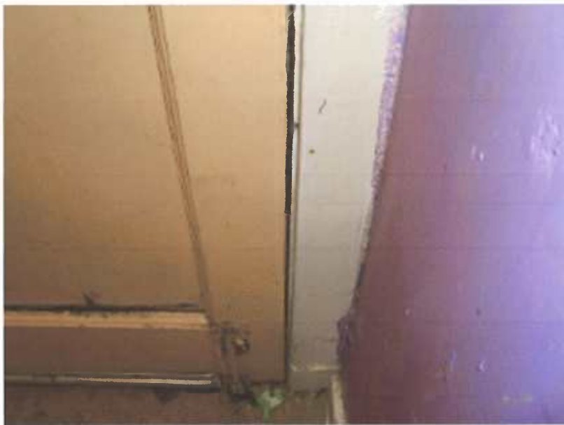
8. REAR DOOR – GAP AT FRAME
