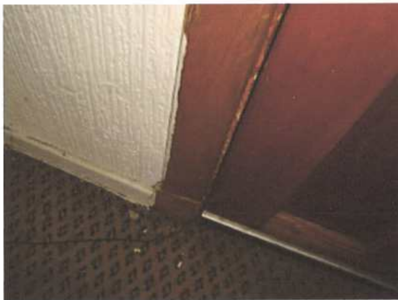
6. FRONT DOOR -- GAP AT FRAME.
