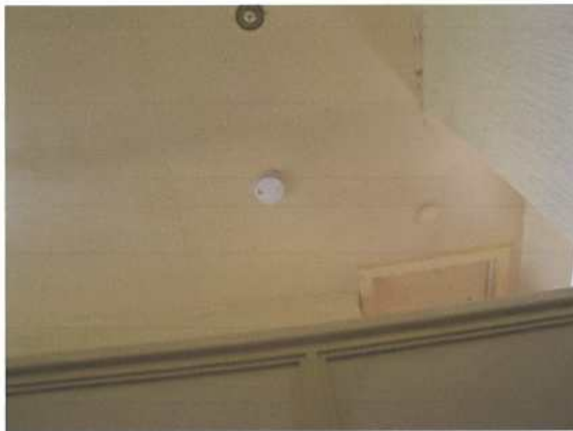
12. UPPER LANDING – SMOKE DETECTOR
