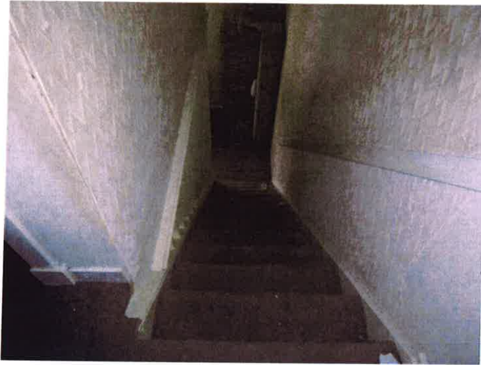
No handrail on steep stair
