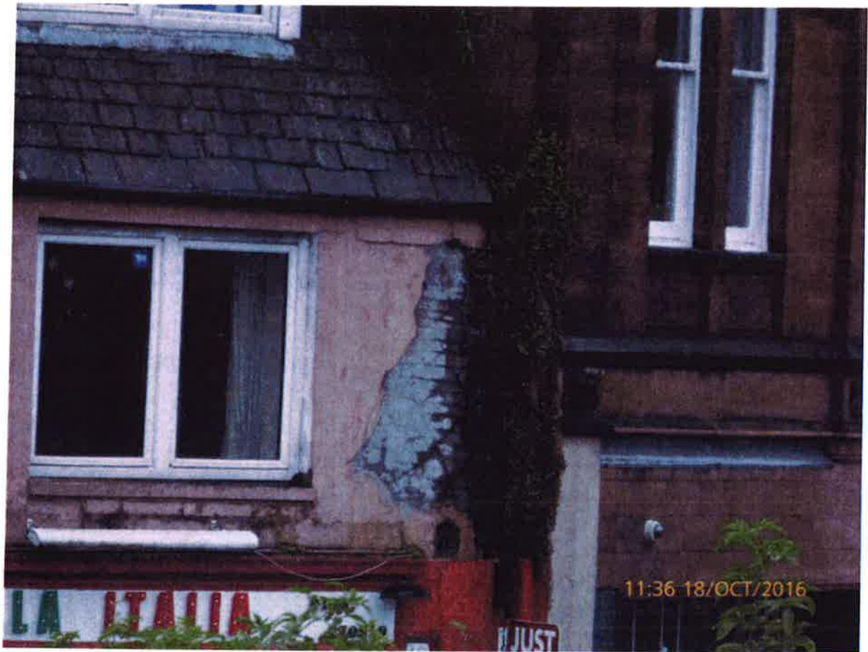
Detail of defective rendering, vegetation and choked downpipe
