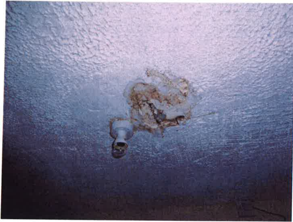
Dampness threat to electric light in bathroom
