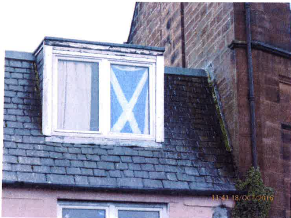
Roof detail showing vegetation and missing flashing
