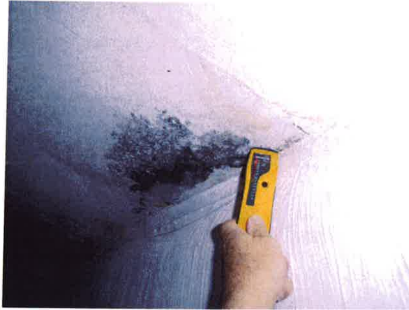
Dampness on ceiling of stairwell
