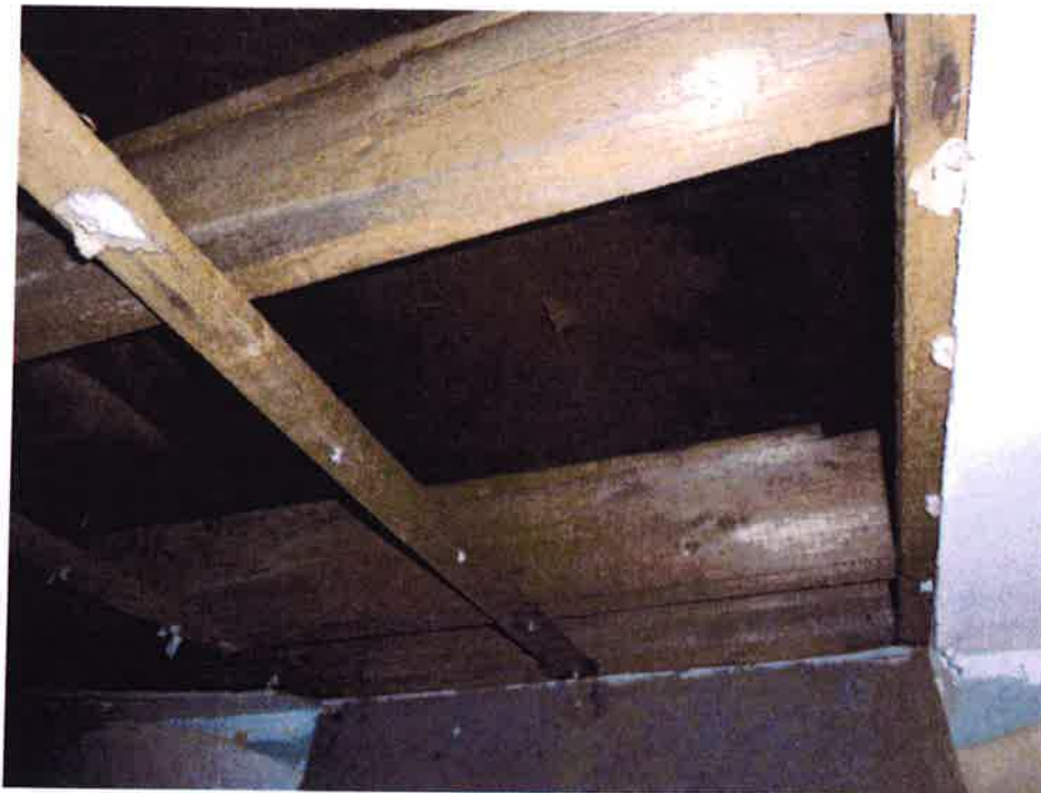
Rainwater penetration and collapsed ceiling in bedroom
