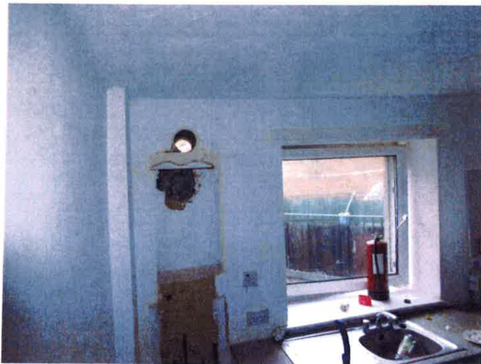
Boiler removed and window not able to be closed
