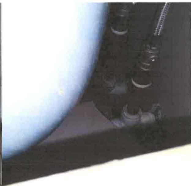
3 View of the unsecured bath trap at the outlet
