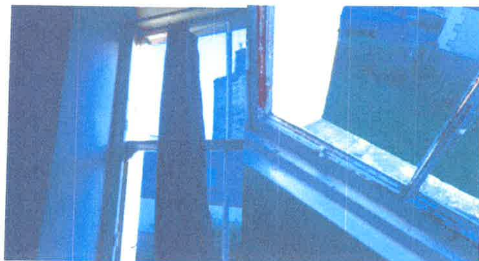
Windows – missing window rope, poor state of repair
