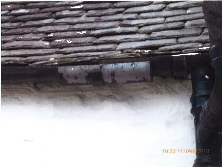
Broken/defective guttering
