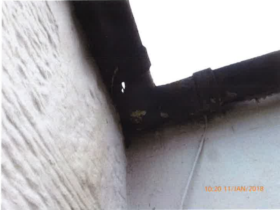
Hole in gutter
