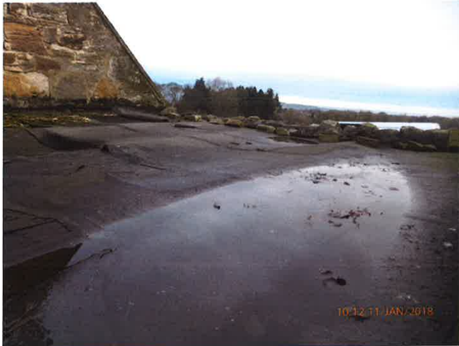
Collapsing flat roof
