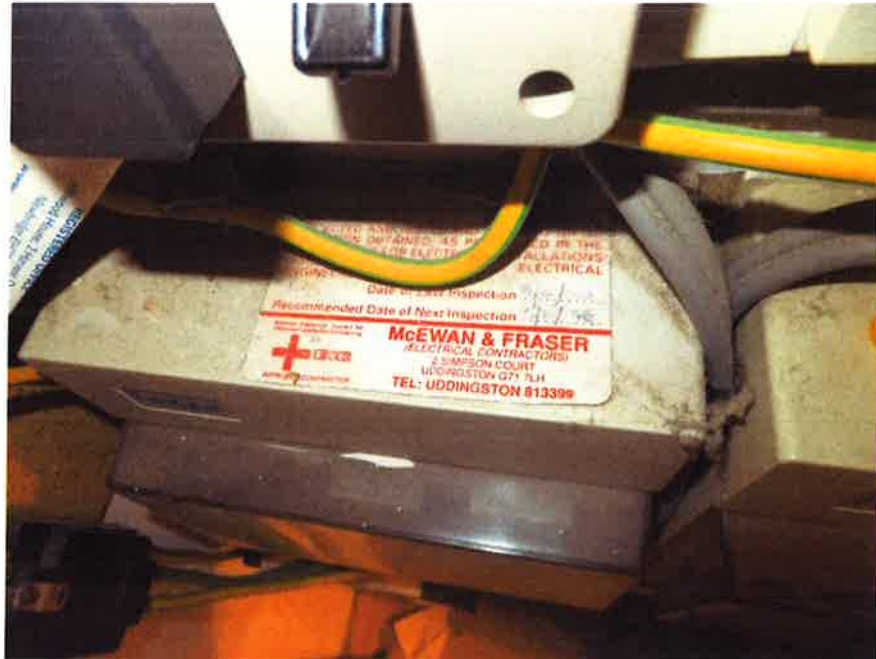
Last test certificate on consumer unit
