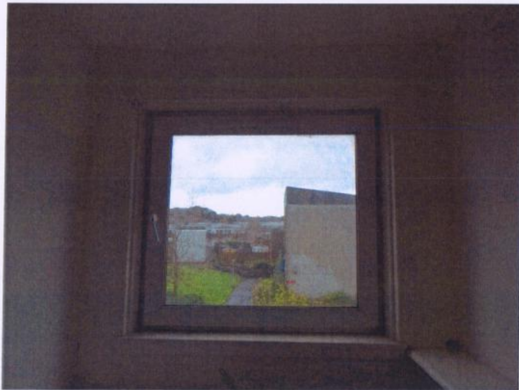
Kitchen utility window hinges are defective and window requires to be lifted to close.
