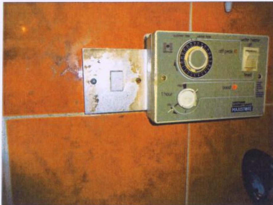
Water temperature was tested in kitchen and bathroom – Lukewarm temperature and poor water pressure noted
