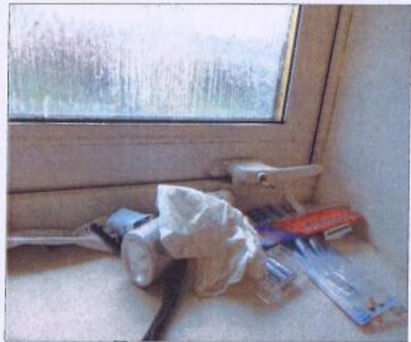
Bathroom window difficult to open and close and unable to lock with key
