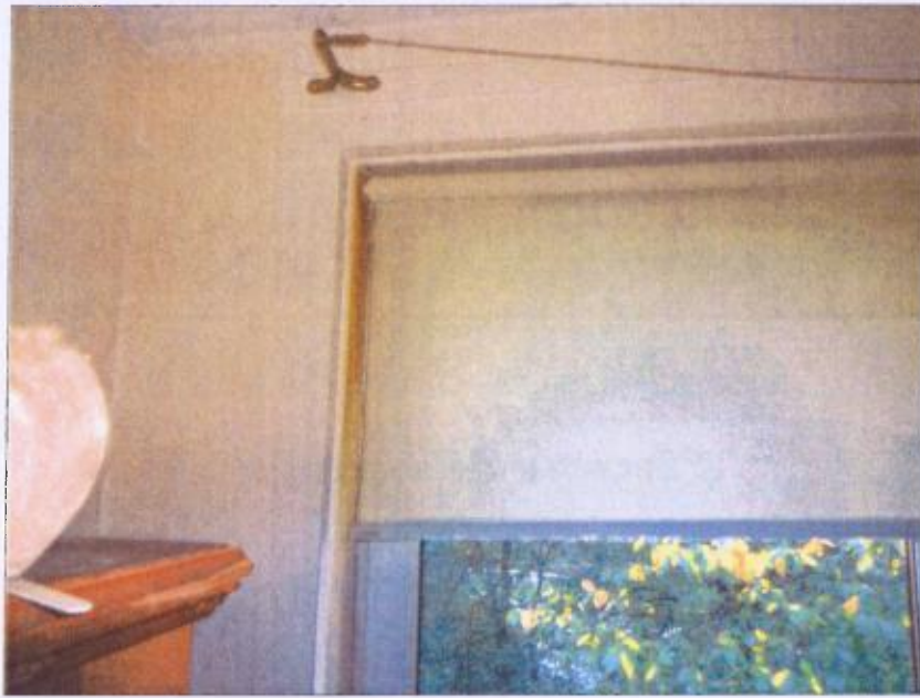
Roller blind preventing window from opening – Main bedroom Unable to lock with key
