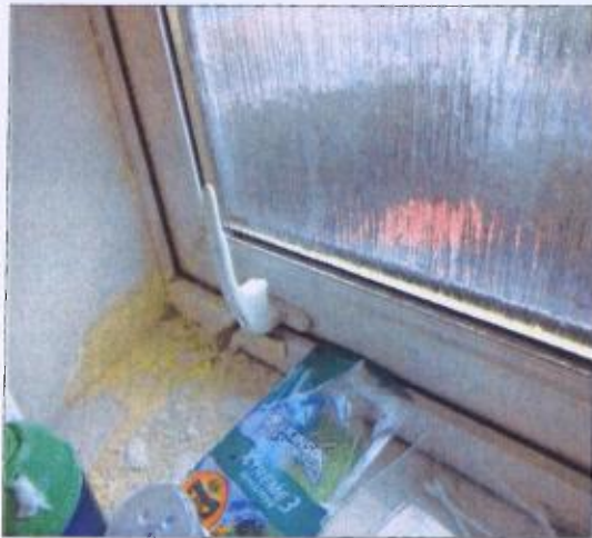
Bathroom window difficult to open and close and unable to lock with key
