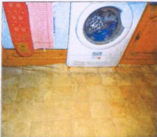
Linoleum in kitchen ripped at washing machine
