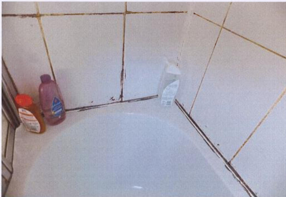
Grouting and mastic to bath
