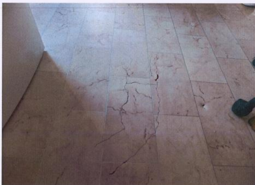
Cracking to kitchen vinyl
