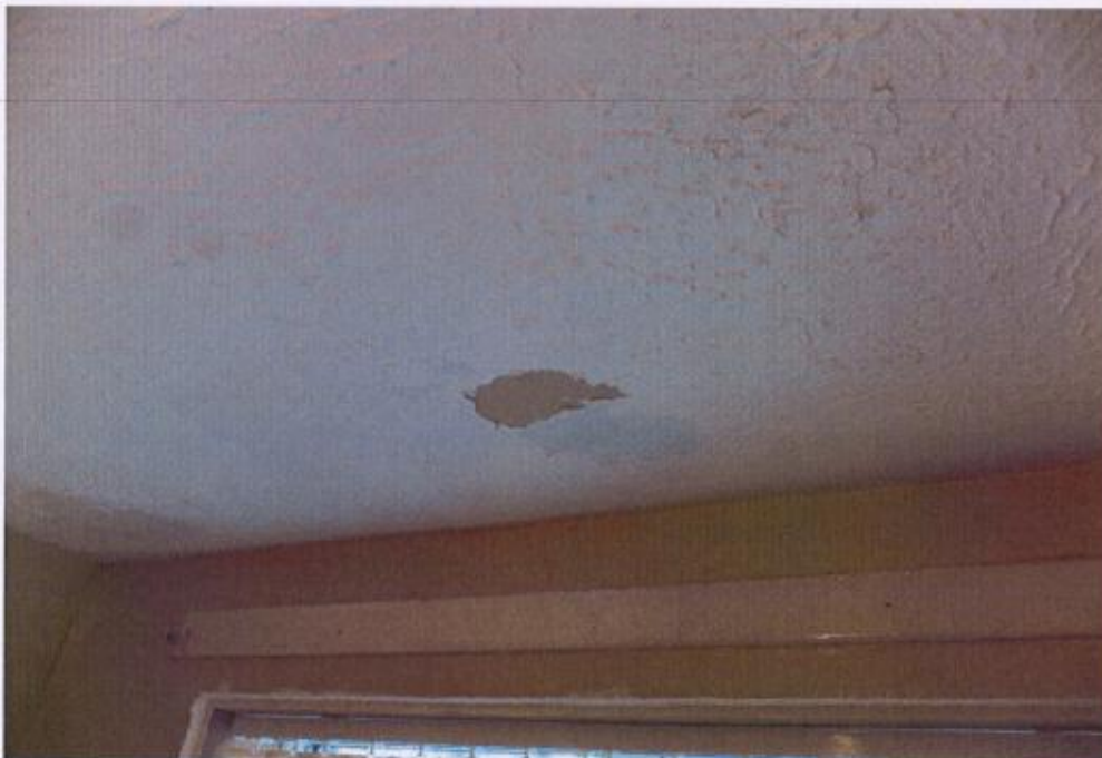
Damaged plaster ceiling
