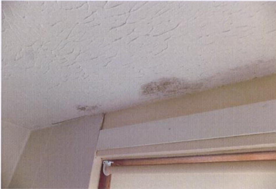
Condensation to ceiling
