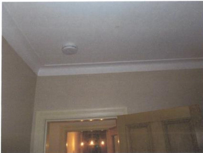
10. Hard-wired smoke detector in living room
