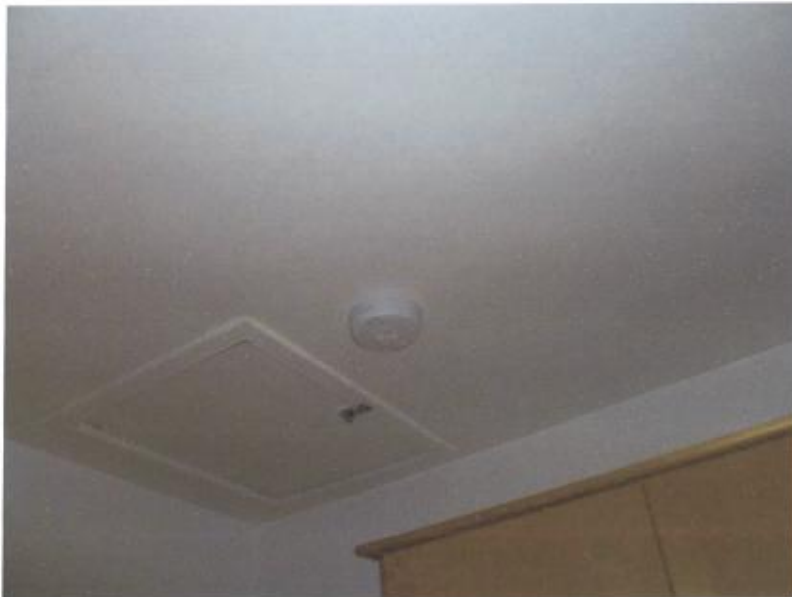
8. Hard-wired heat detector in kitchen
