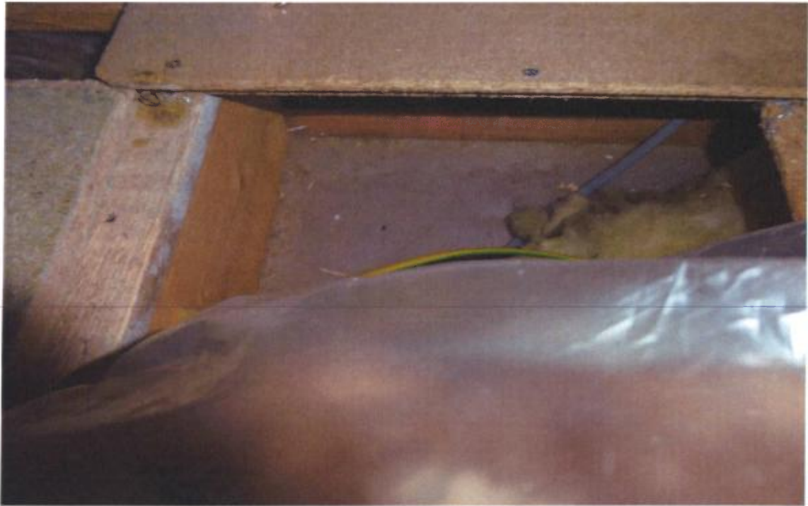
Loft insulation missing from beneath boarding
