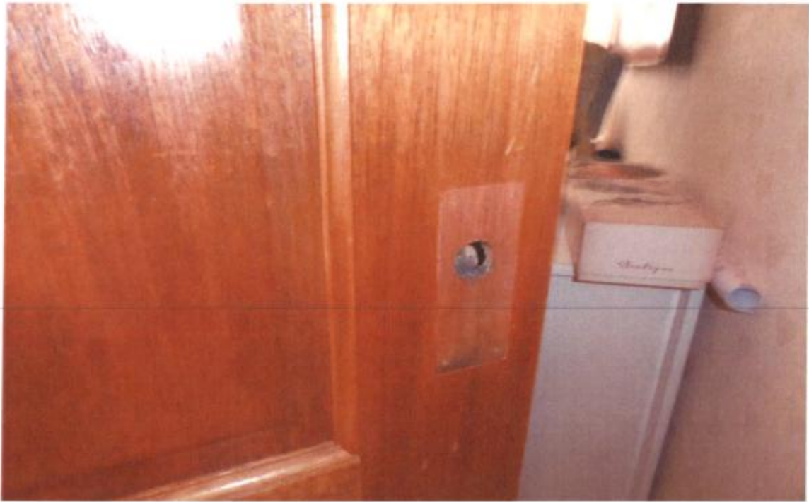
Spare bedroom door with missing handle and latch
