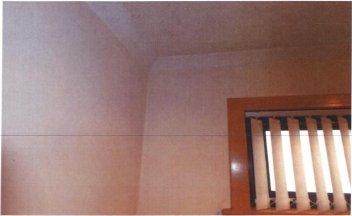
Ceiling and upper wall discoloured by water damage from leaking water pump in loft
