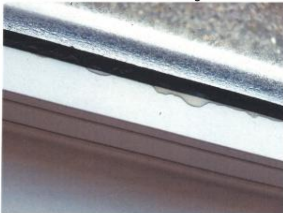
13 Internal condensation to window pane.
