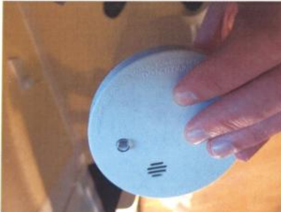
1 Unfixed battery operated smoke detector (1 No. within property).
