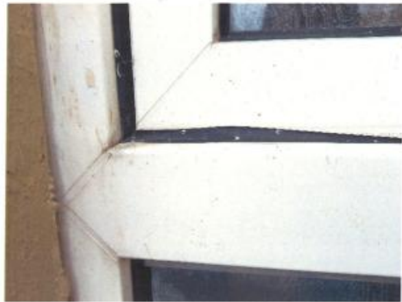
8 Weatherproof strip defective – view of rear elevation window.
