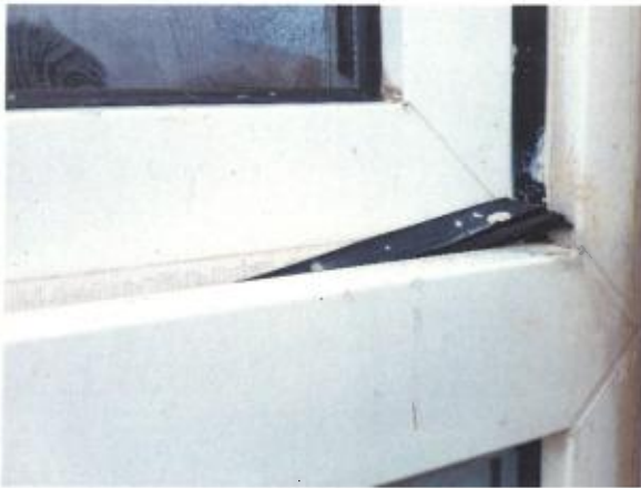
7 Weatherproof strip defective – view of rear elevation window.
