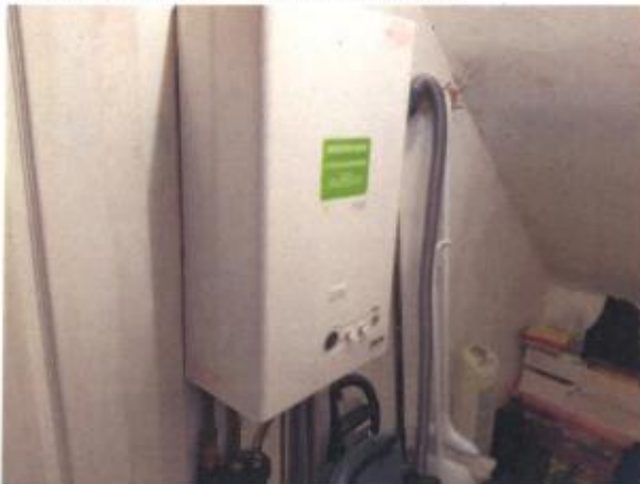
5 Gas fired boiler.
