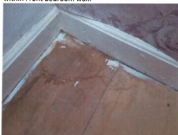
19 Carpet taken back and evidence of water staining at corner.
