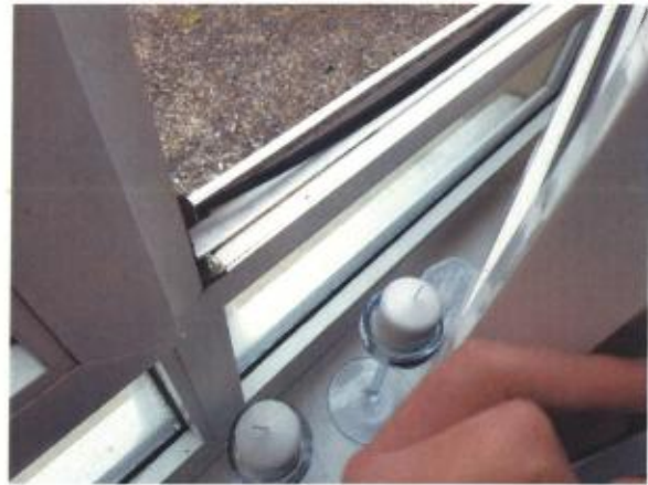
10 View of loose weatherstrip viewed internally.
