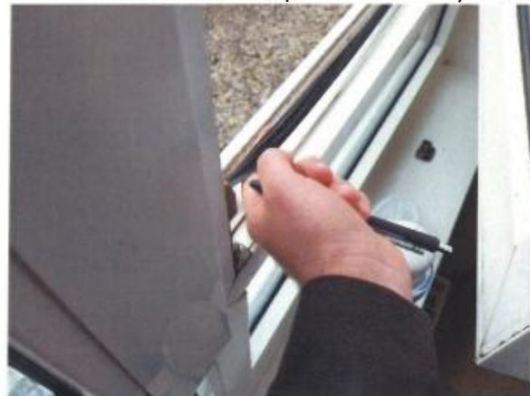
14 Loose weatherseal not adhered.
