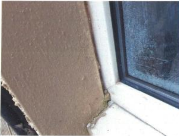
9 Seal between window frame and ingoe.
