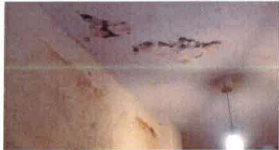
Photo 5 – Water damage on kitchen ceiling
