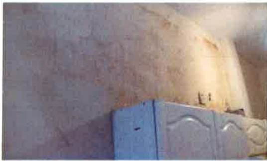
Photo 2 – Water damage on kitchen wall
