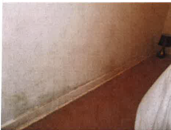
Bedroom - black spot mould accumulation on wall and skirting adjacent to wardrobe
