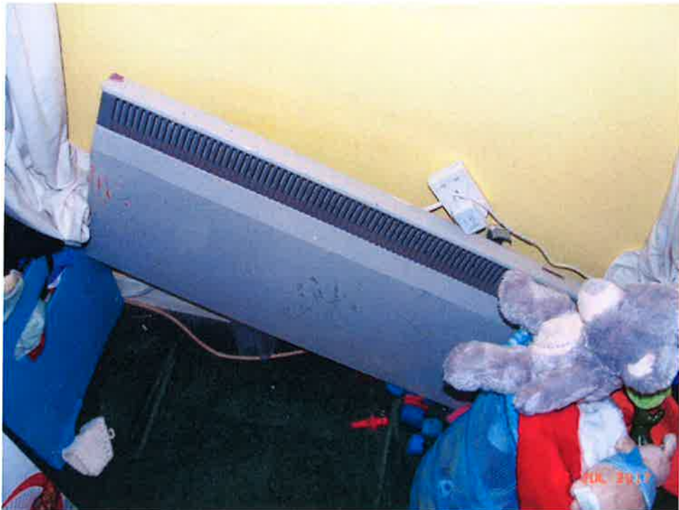
Back Bedroom wall heater loose from wall
