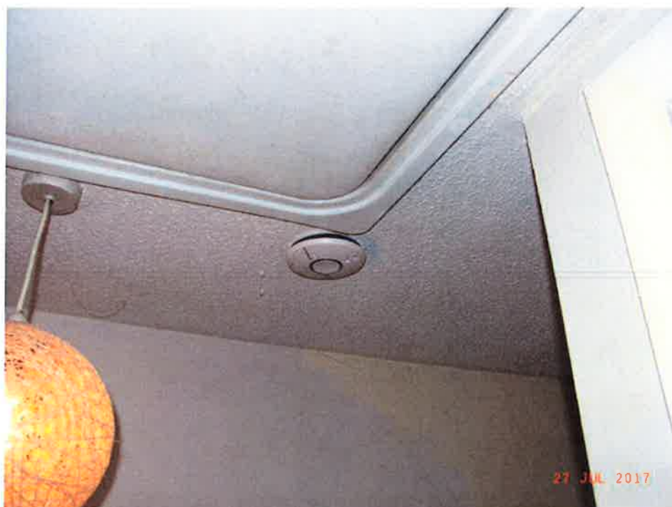
Battery powered smoke detector in Landing
