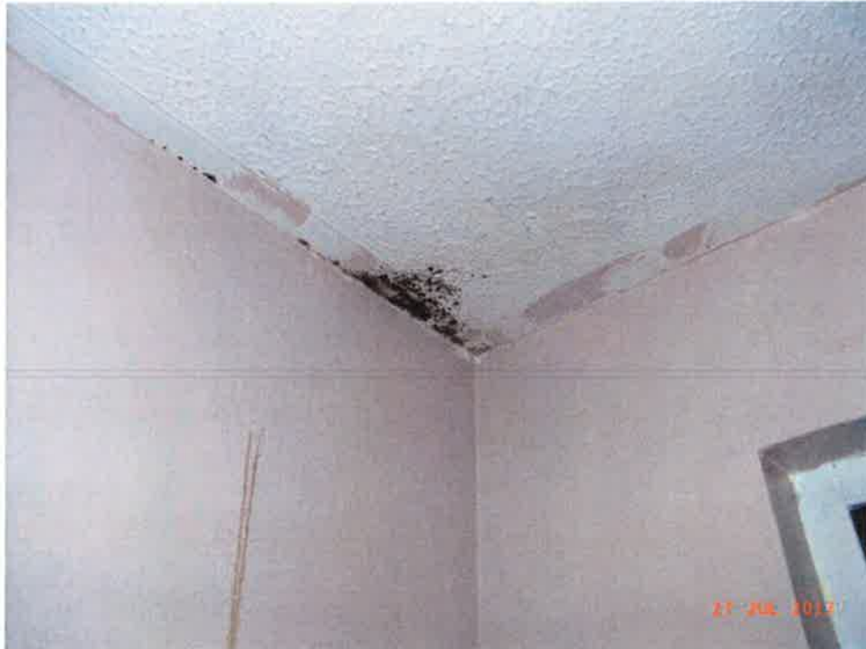
Condensation mould to Entrance Vestibule ceiling (2)
