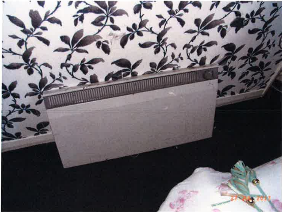
Front Bedroom wall heater loose from wall
