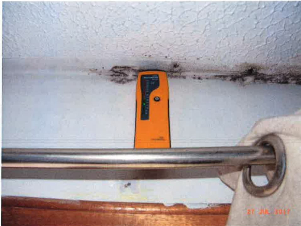
Condensation mould to front Bedroom ceiling (2)
