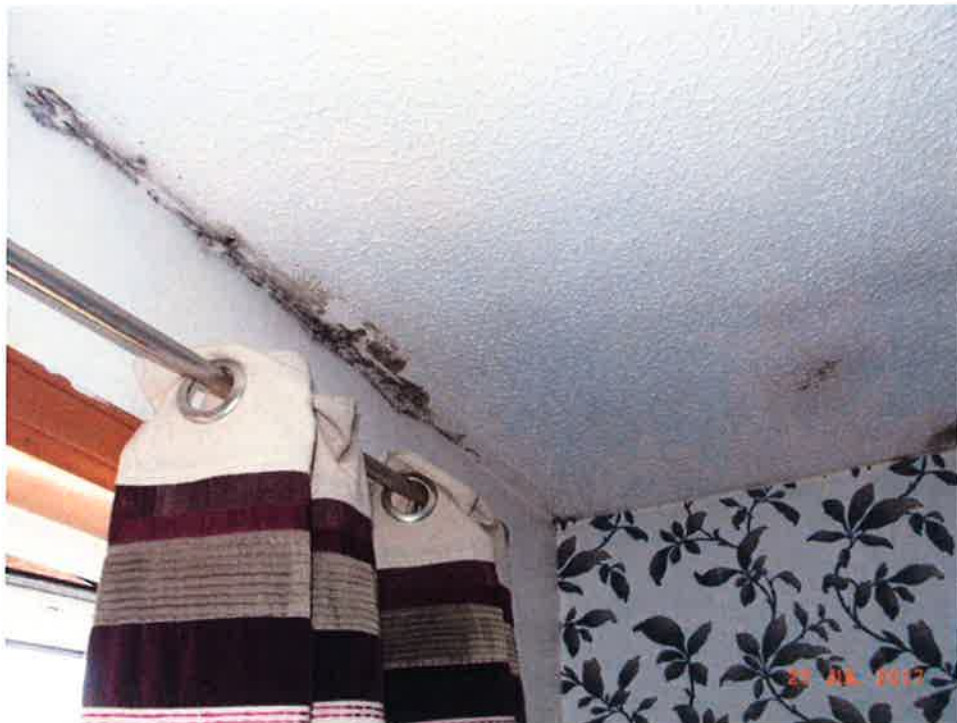
Condensation mould to front Bedroom ceiling (1)
