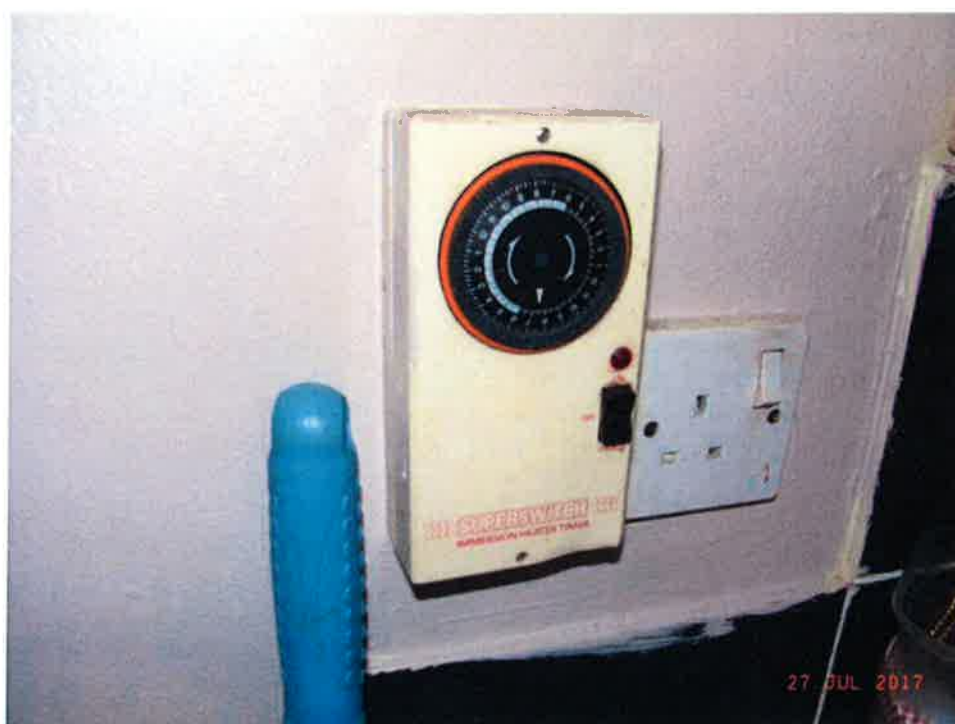
Electric Immersion Heater switch in Kitchen
