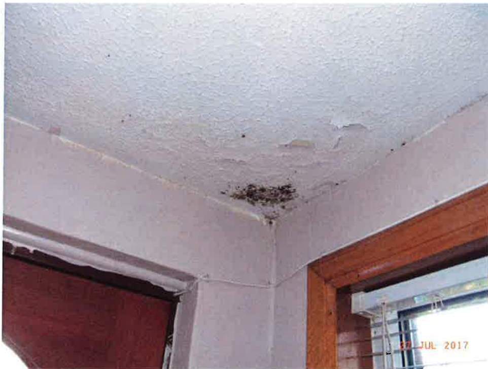
Condensation mould to Entrance Vestibule ceiling (1)
