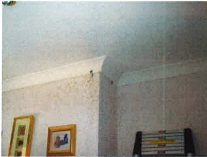
Staining at chimneybreast in Living Room
