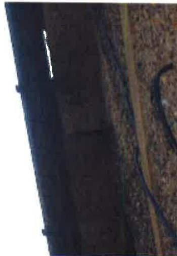
Gap between roof and gutter at front elevation
