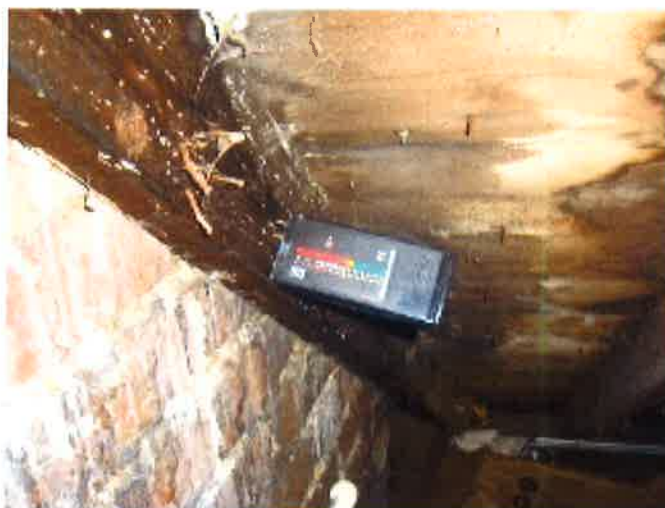
“Red” damp meter reading in rafter adjacent to chimneyhead in roof void
