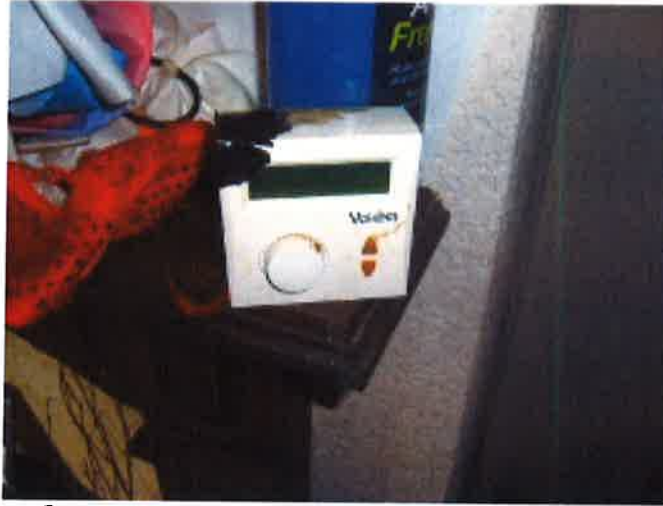
Central heating timeclock/thermostat
