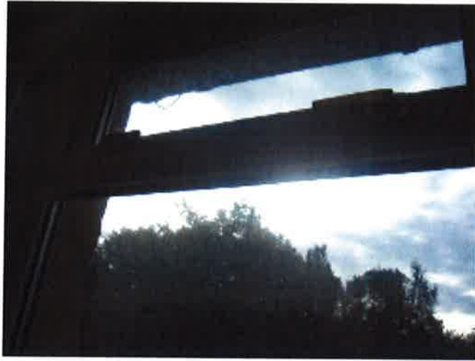
Missing window handle catches in Living Room
