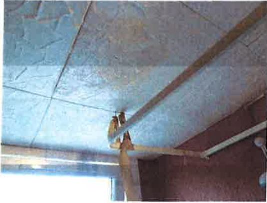
Photograph 7:- Residual damp staining and temporary shower rail support
