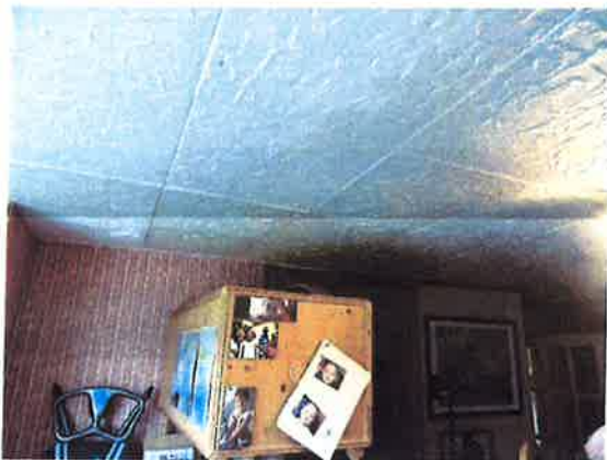
Photograph 11 Polystyrene ceiling tiles kitchen area
