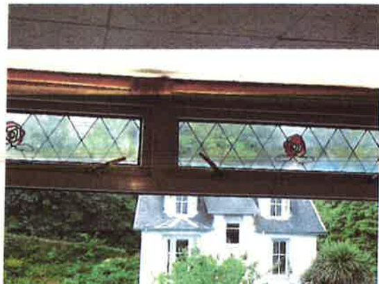
Photograph 10:- Failed seals at kitchen window hoppers.
