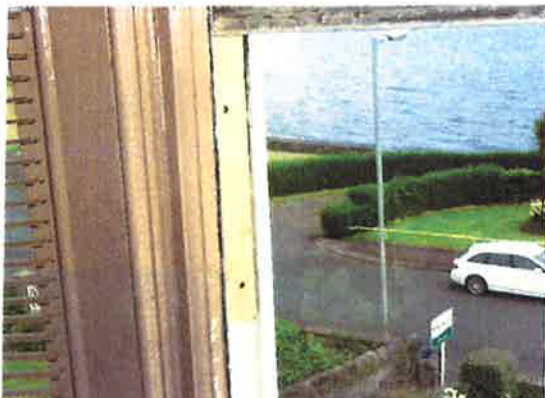
Photograph 5:- Temporary external timber support living room window.
