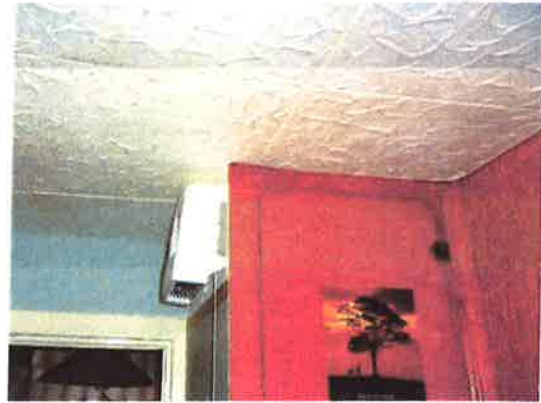
Photograph 8:- Polystyrene ceiling tiles and wall hung bathroom warm air heater
