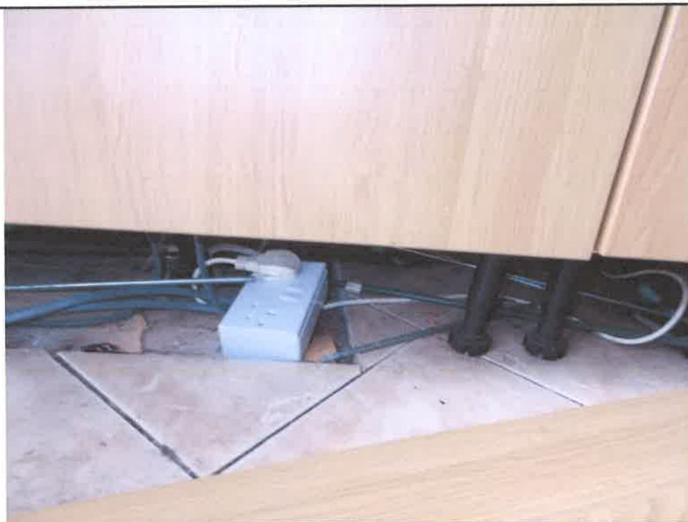
13. Electric Socket outlet below unit in Kitchen
