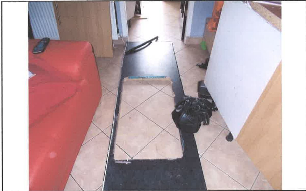
9. Stripped out Worktop with sink cut out
