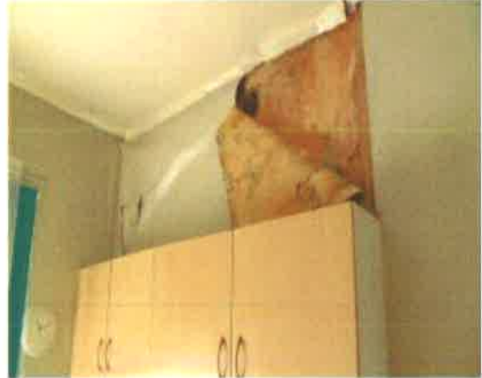
(Ph5) Previous water damage + wall vent
