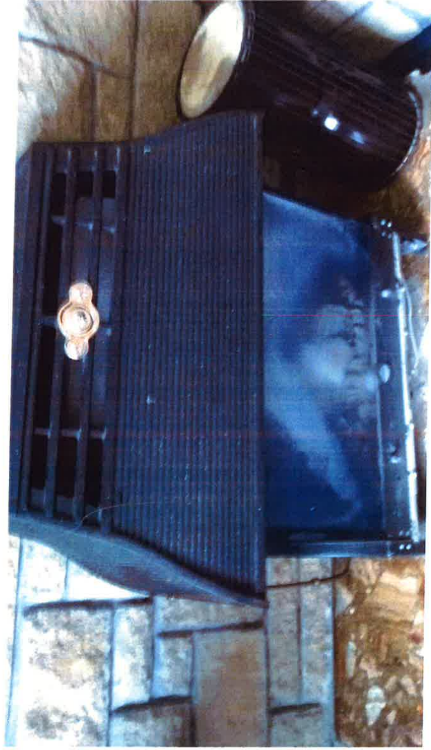
Sitting room appliances: gas fire disconnected
