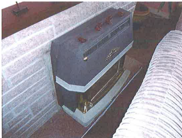
2. Gas fire with back boiler
