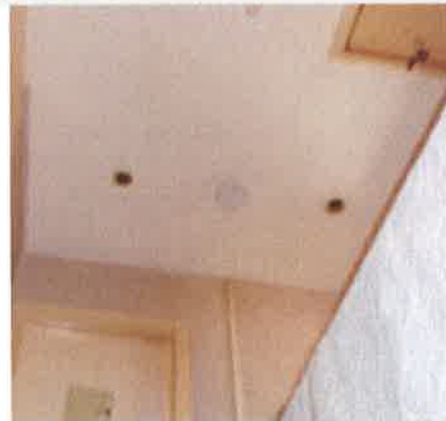
Landing - ceiling mounted smoke alarm
