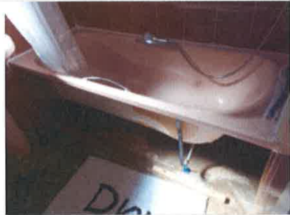
Bathroom showing missing bath panel
