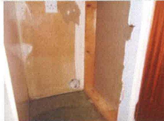
Tumble dryer vent - exposed hole packed with paper - internal view
