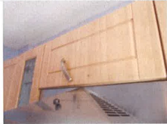
Kitchen - showing defective/loose handle to unit above cooker hood
