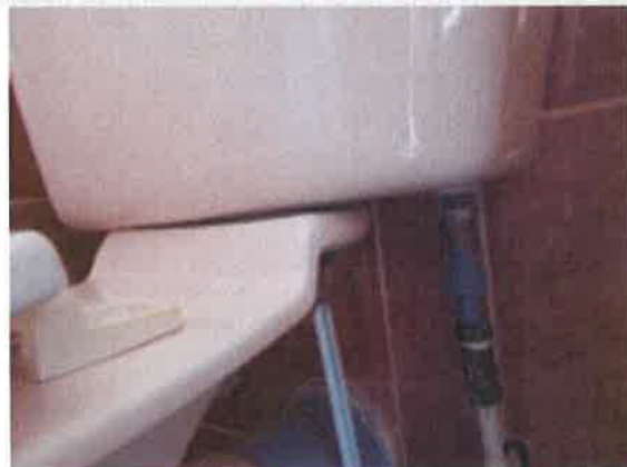
Bathroom - showing uneven gap between cistern and toilet bowl
