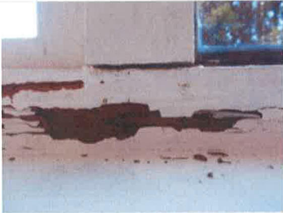
Living Room window- internal - showing rot
