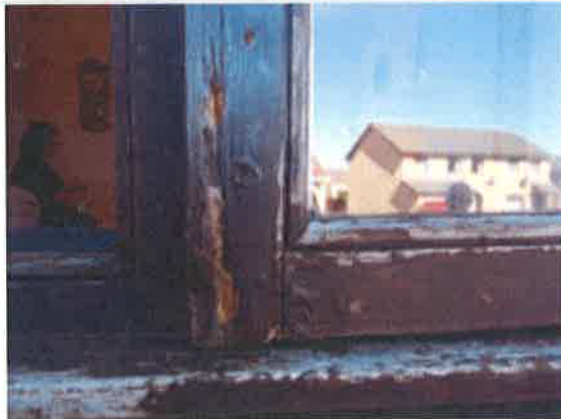
Living Room window - external - showing rot and broken/missing external pane to centre window double glazing
