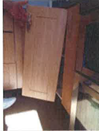
Kitchen - showing defective/loose hinges to corner base unit
