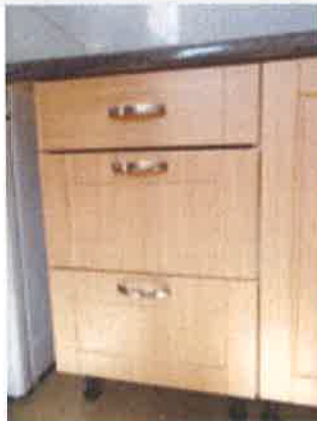
Kitchen - showing gap at doors to drawer
