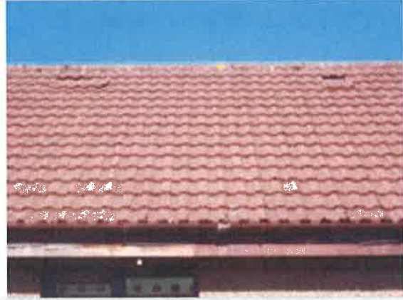
Roof - rear pitch - 3 roof tiles dislodged
