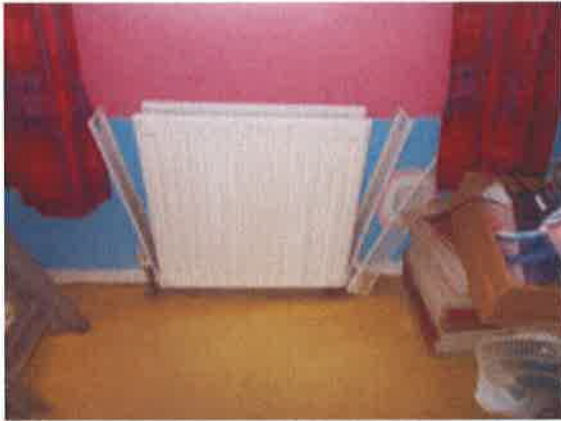
Front bedroom right side - radiator not secured to right side bracket and loose side panels
