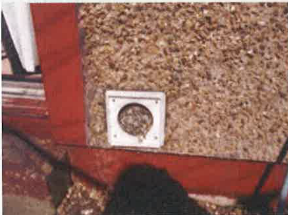
Tumble dryer vent - missing cover/hole packed with paper - external view
