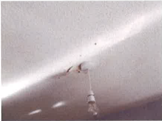
Kitchen - ceiling damaged by leak from bathroom
