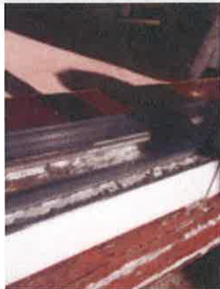
Patio Door showing broken/missing external pane to double glazing
