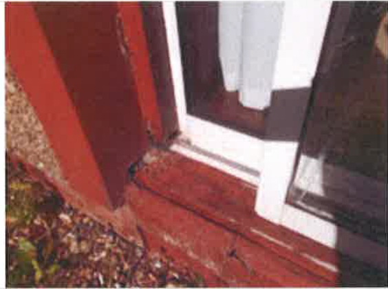
Patio doors showing one door not secure on the track and rot to external timber sill
