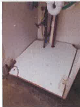
Kitchen sink base unit - dilapidated/water damage and missing door
