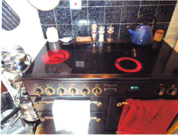
Photograph 1 :- Cooker hob with defective front right inner ring.
