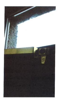
Patio doors – handle fixed but doors are difficult to open/close and locks misaligned and damaged
