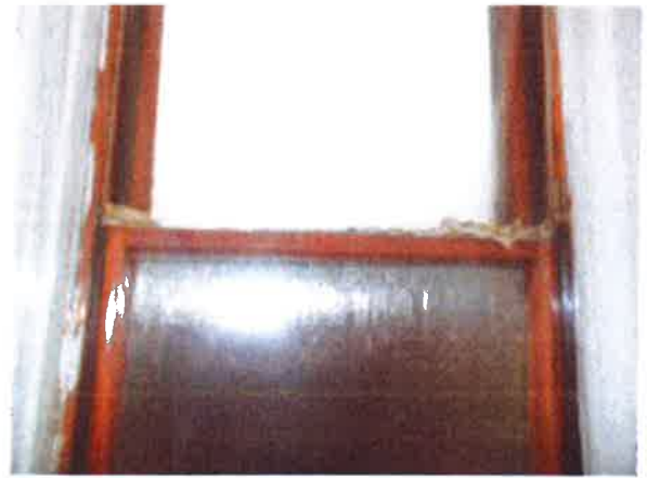
Bathroom Window - kitchen towel used to block draughts/plastic sheet covering entire internal surface
