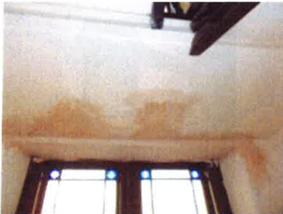
Middle landing - plaster to ceiling above window patched.
