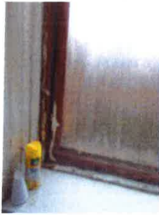
Bathroom Window - kitchen towel used to block draughts/plastic sheet covering entire internal surface
