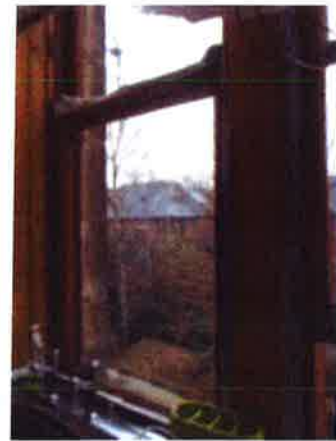
Kitchen window - left side - towels on top rail of lower sash and not possible to open.
