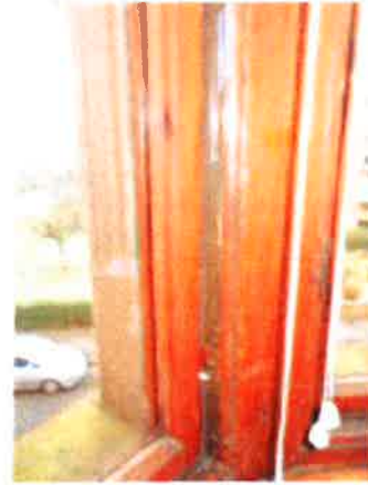
Living Room - Bay Window - left side - showing tape applied by tenant to block draughts
