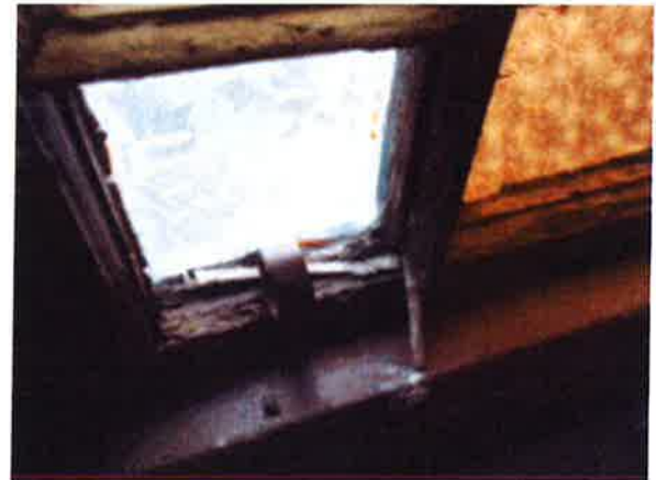
Top landing - close window showing rot
