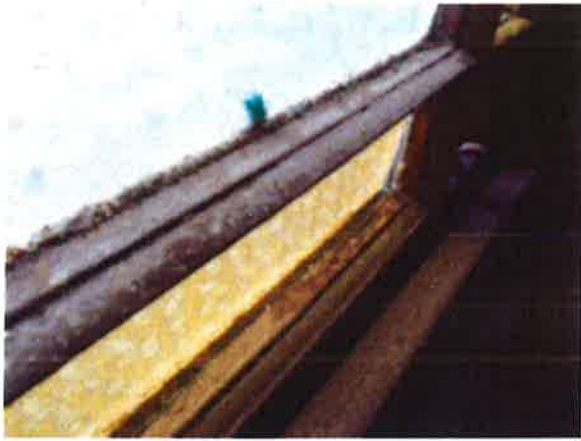
Top landing window - loose lower sash/missing cords.
