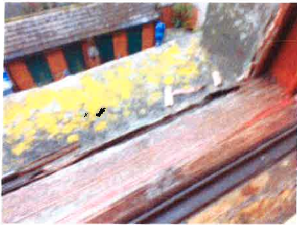
Kitchen Window - right side - rot to external sill
