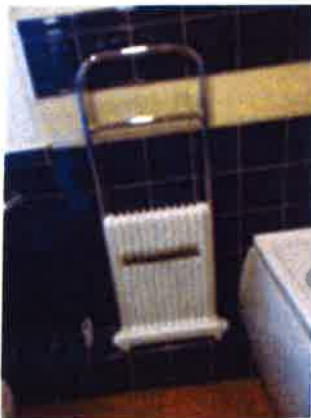
Bathroom - electric heater and towel rail
