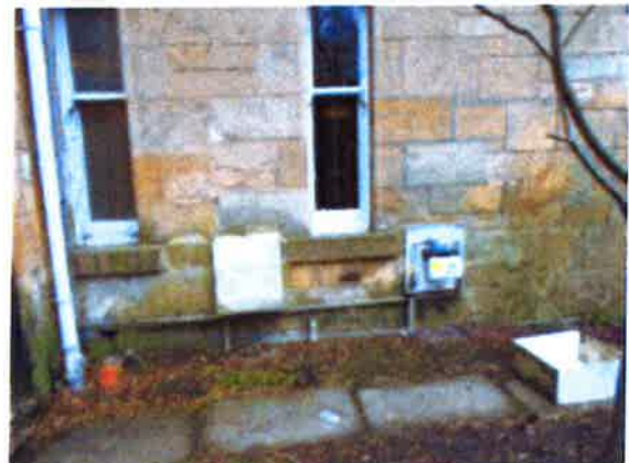
Exterior walls and built up ground level - Small Bedroom - hip end
