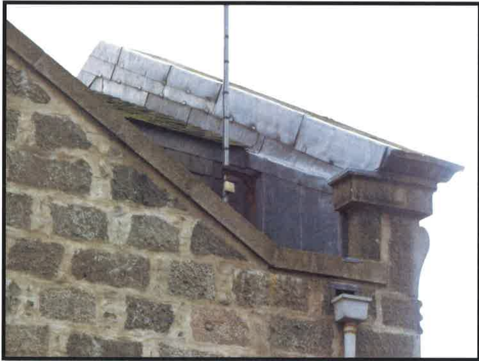
Figure 9 Rear of Crown Street pediment
