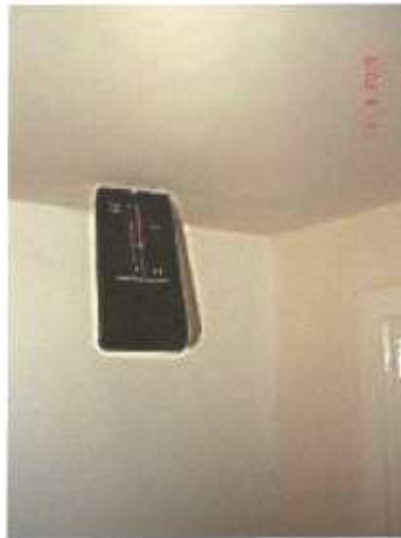
Meter reading on ceiling
