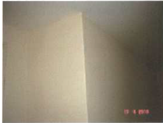
Living Room Ceiling
