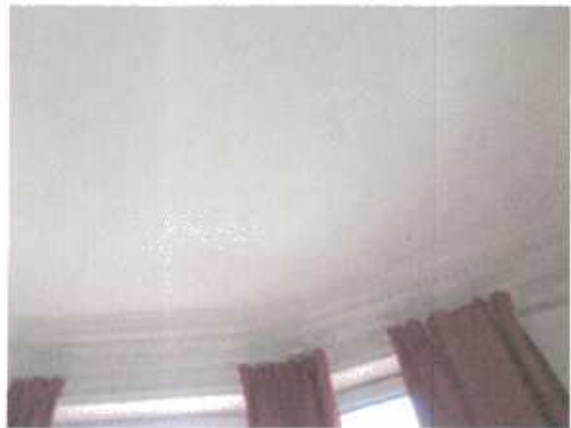
Living Room ceiling over bay window
