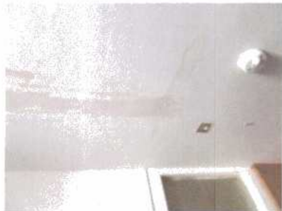
Kitchen ceiling towards door opening
